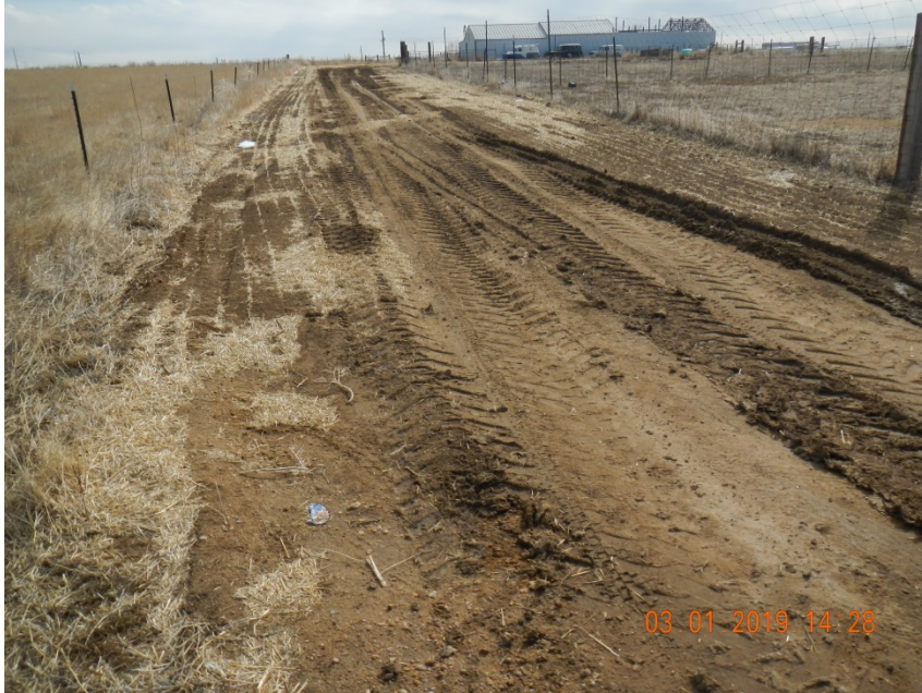
Photo 1. Photo taken from the access road, facing South. Appears the Operator recently completed reclamation activities with drill seed rows and straw crimped mulch.
