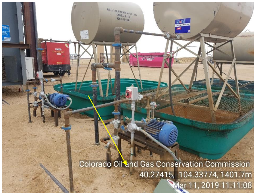
Photo 13 Stained soil under transfer pump for motor oil
