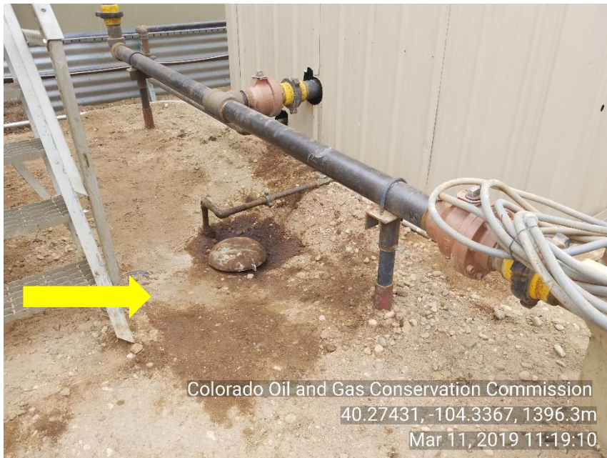
Photo 29 Stained soil out side of lact building around what appears to be buried vault.
