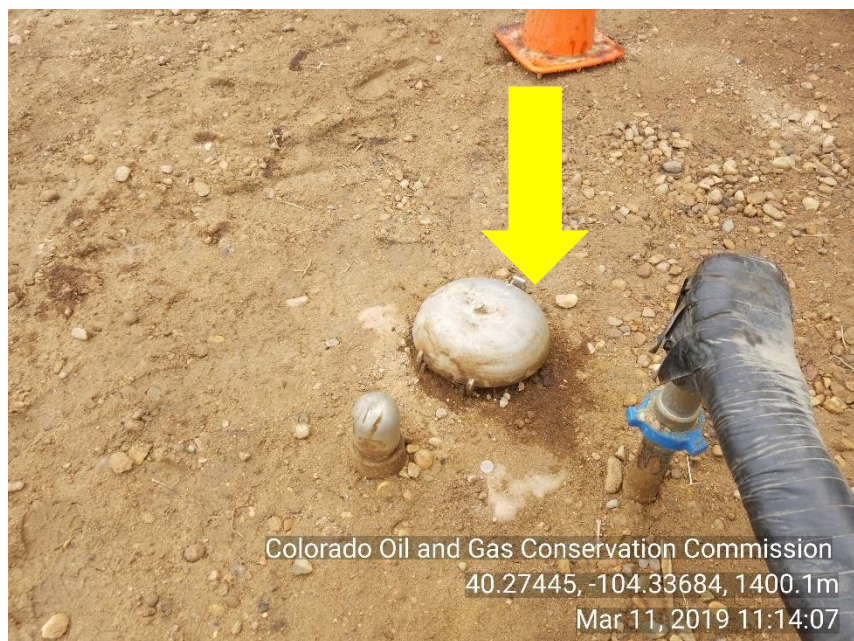
Photo 19 stained soil around lid of what appears to be buried vault out side containmet wall.
