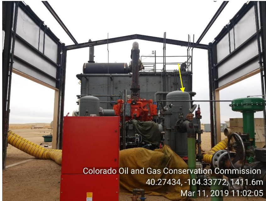
Photo 5 Gas compressor Pic. Tarps and hoses from heaters
