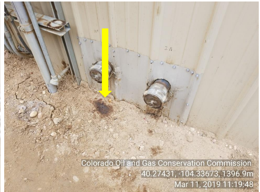
Photo 30 stained soil outside lact building out side of crude oil containment
