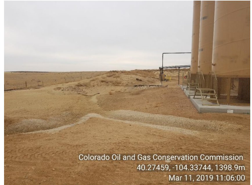
Photo 12 location drainage and sediment trap
