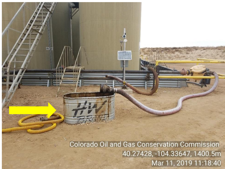
Photo 27 Improper storage of load line hoses. No secondary containment under oil container.
