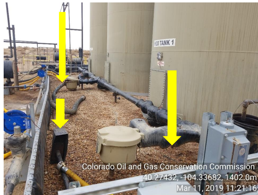
Photo 34 stained soil under load out lines, trash(mailbox) and improper storage of houses.
