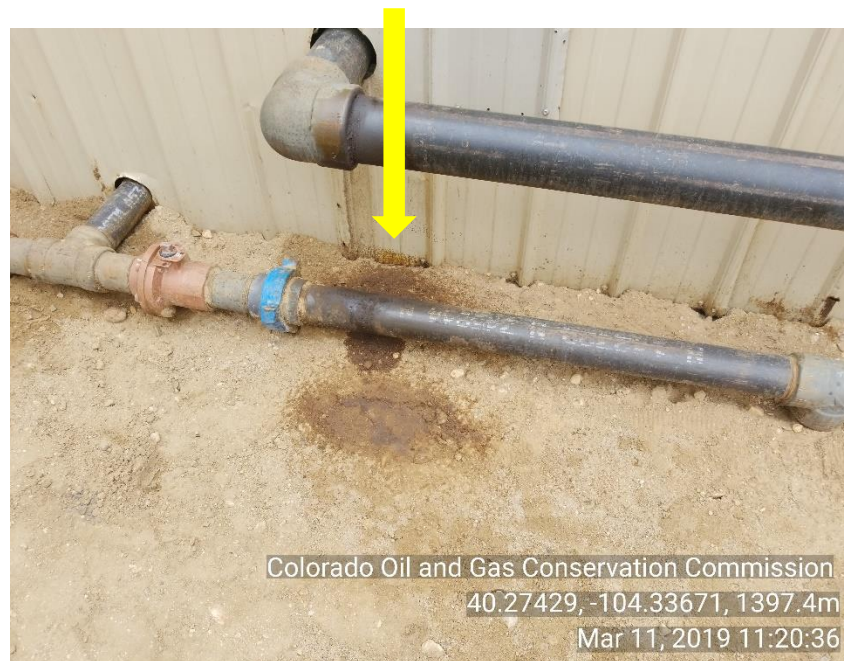
Photo 32 stained soil outside lact building out side of crude oil containment
