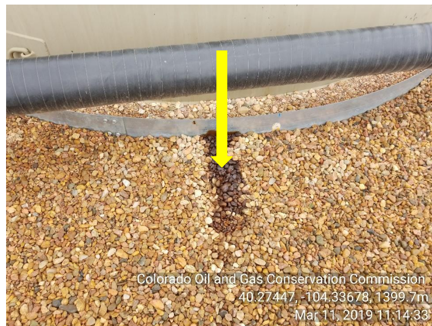
Photo 20 Stained soil around grade ring of crude oil tank inside containment
