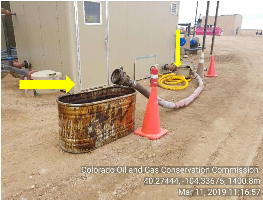
Photo 23 Improper storage of hose's and no secondary containment under oil container
