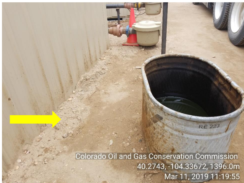
Photo 31 Unused equipment and not on secondary containment
