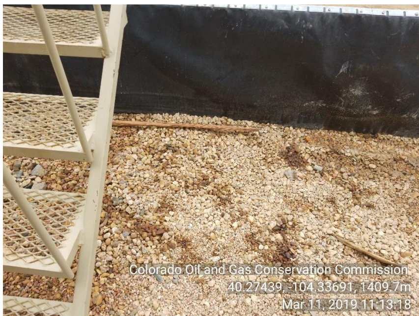
Photo 17 stained soil inside crude oil containment
