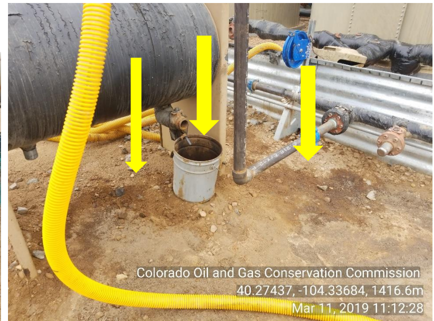
Photo 14 Stained soil under and around Knock out tank in front of TNK BTRY. 5 gal bucket is trash
