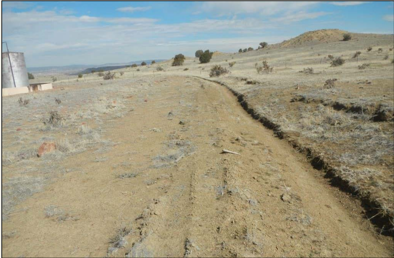
Photo 8. View of stormwater diversion for run-on control along the eastern edge of the project area. Does not appear sufficient to divert stormwater flows from significant runoff events.
