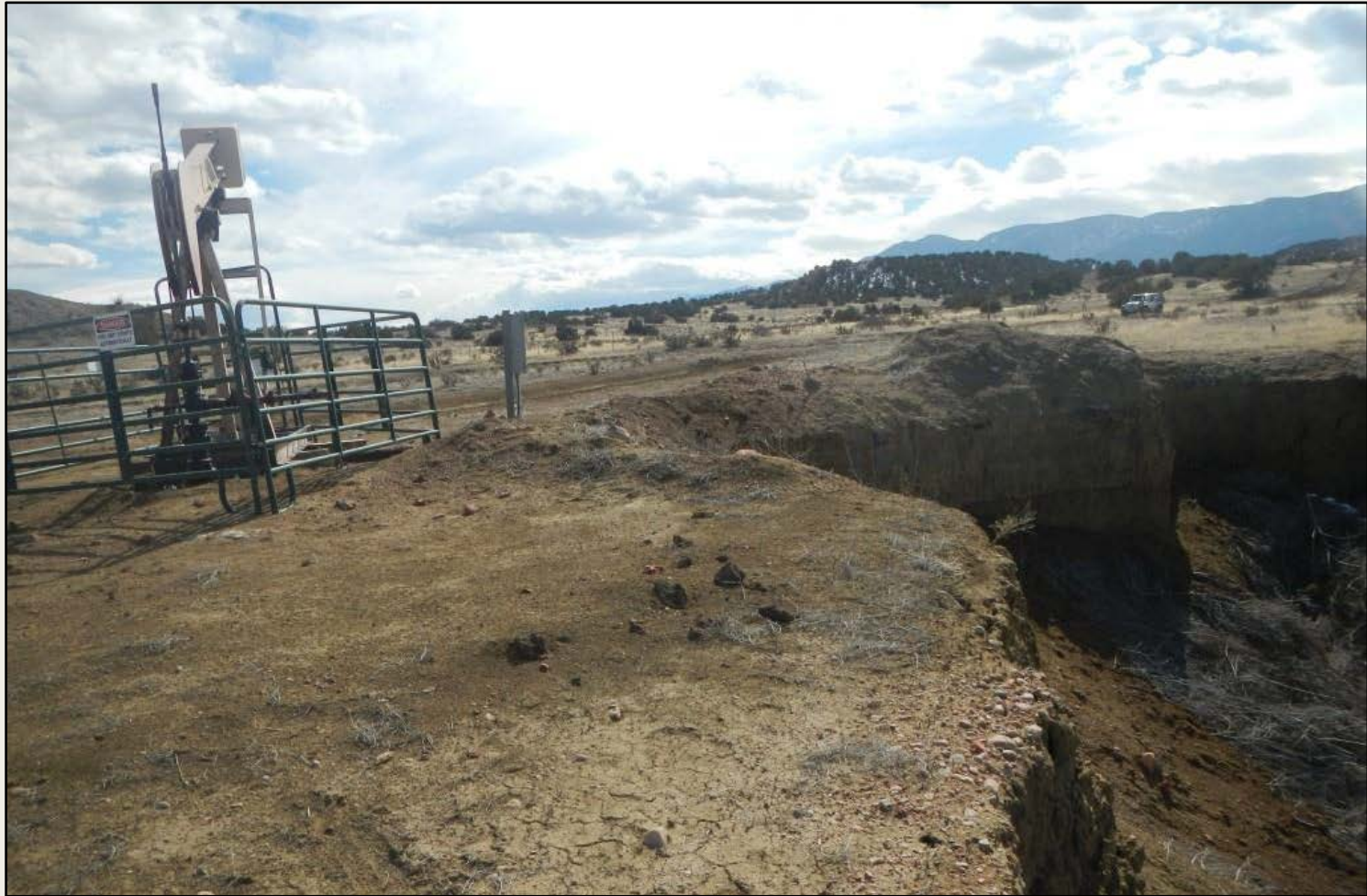
Photo 1. View of the western project area from the western edge facing southward. Wellhead is adjacent to an erosion channel. This area needs immediate stabilization to prevent any further erosion.
