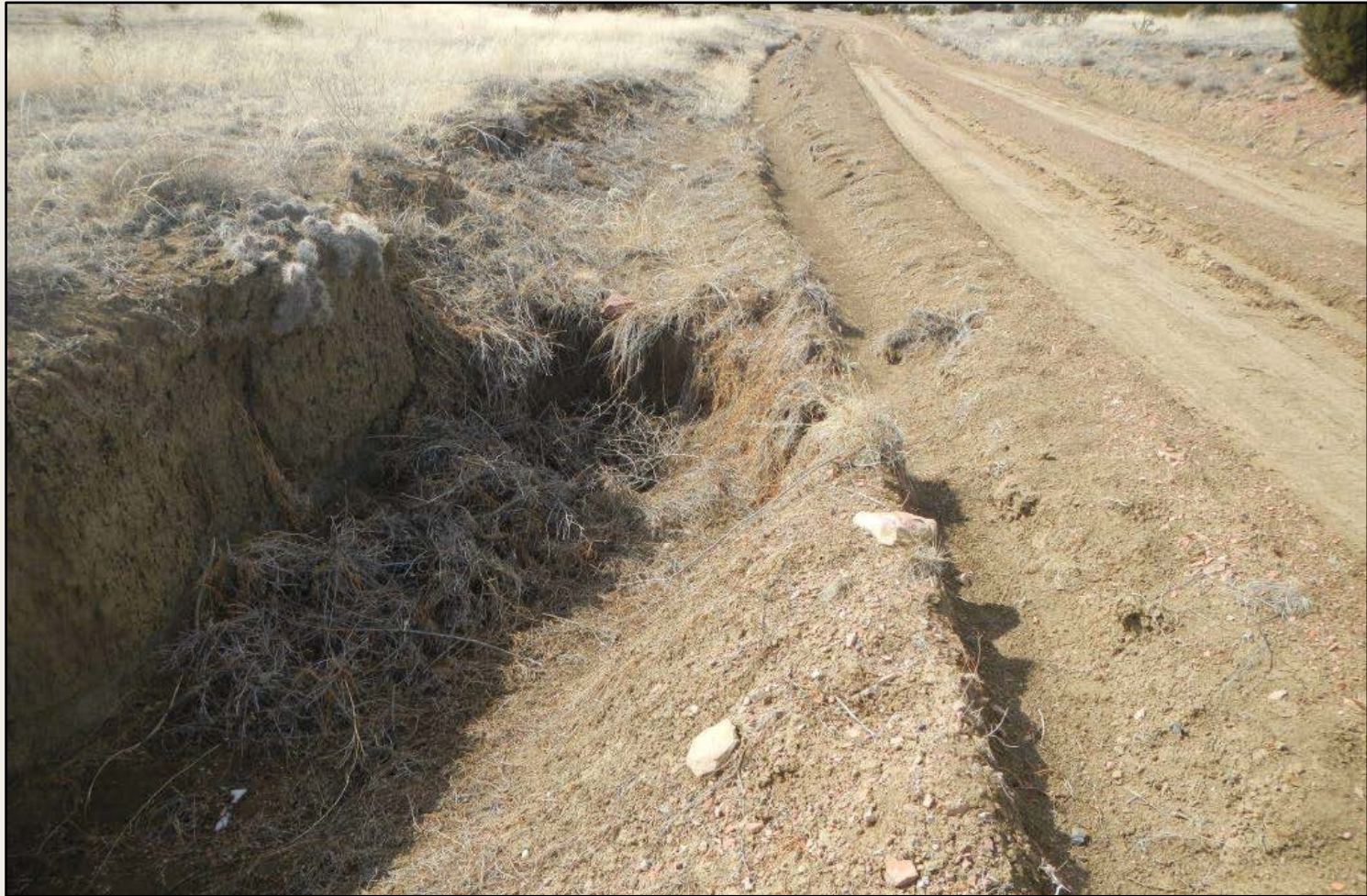
Photo 9. View of erosional headcut, approximately 3 feet wide and deep, along the eastern edge of the access road. Stormwater controls are needed to stabilize erosion within the roadside ditches.
