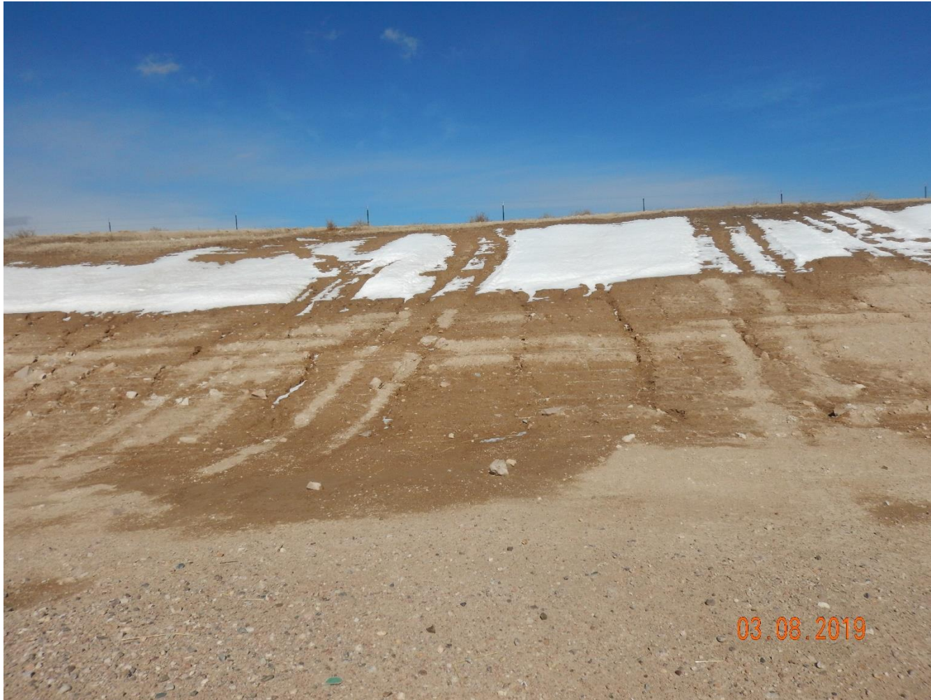
Photo 25: See comments under photo 23. Photo also shows tracks left by a vehicle that appears to have been traveling upon the slopes and ditch of the location. This does not comply with surface disturbance minimization. Vehicle travel may also be contributing to erosion degradation of the pad.
