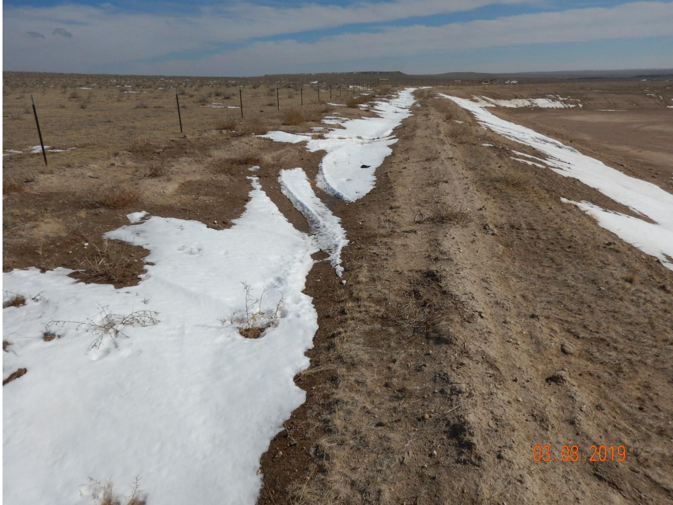
Photo 8: Photo taken from the ditch of the north end of the location, facing east. Photo shows tracks left by a vehicle that appears to have traveled upon the slopes and ditch of the location. This does not comply with surface disturbance minimization.
