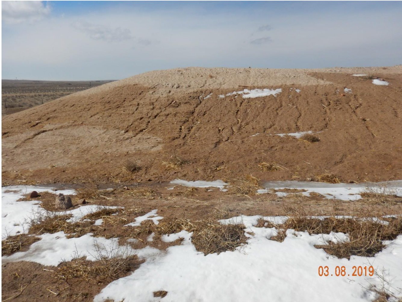
Photo 15: Photo taken from the southeast corner of the pad, facing west. Photo shows stormwater erosion degradation on the slopes of the pad.
