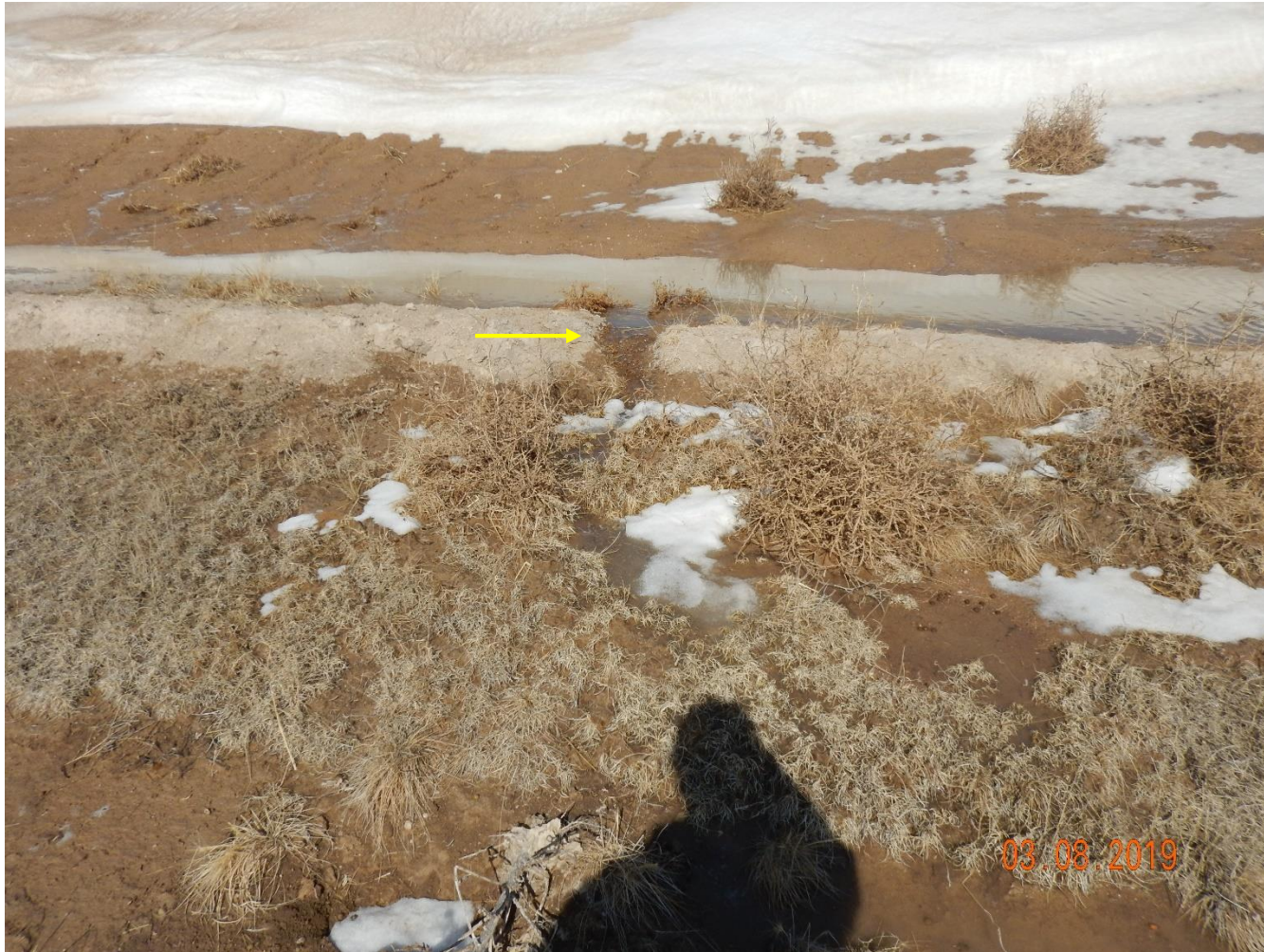
Photo 17: Photo taken from the stormwater ditch on the south end of the location. Photo shows section of the ditch that appears to have filled with sediment allowing stormwater to breach the BMP and discharge from location.
