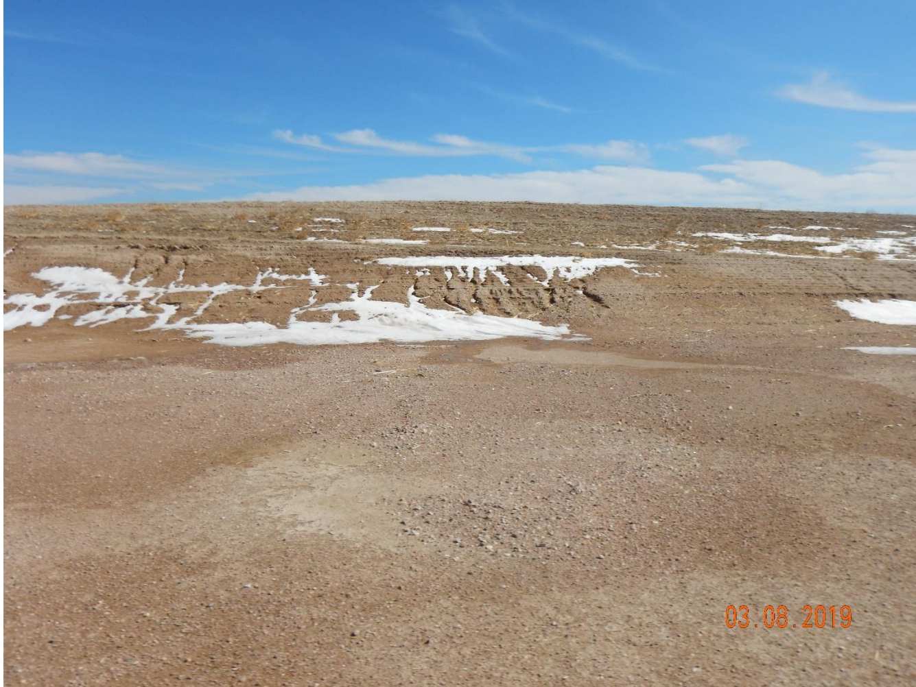
Photo 26: Photo taken from the east end of the pad, facing east. Photo shows erosion degradation at the topsoil stockpile.
