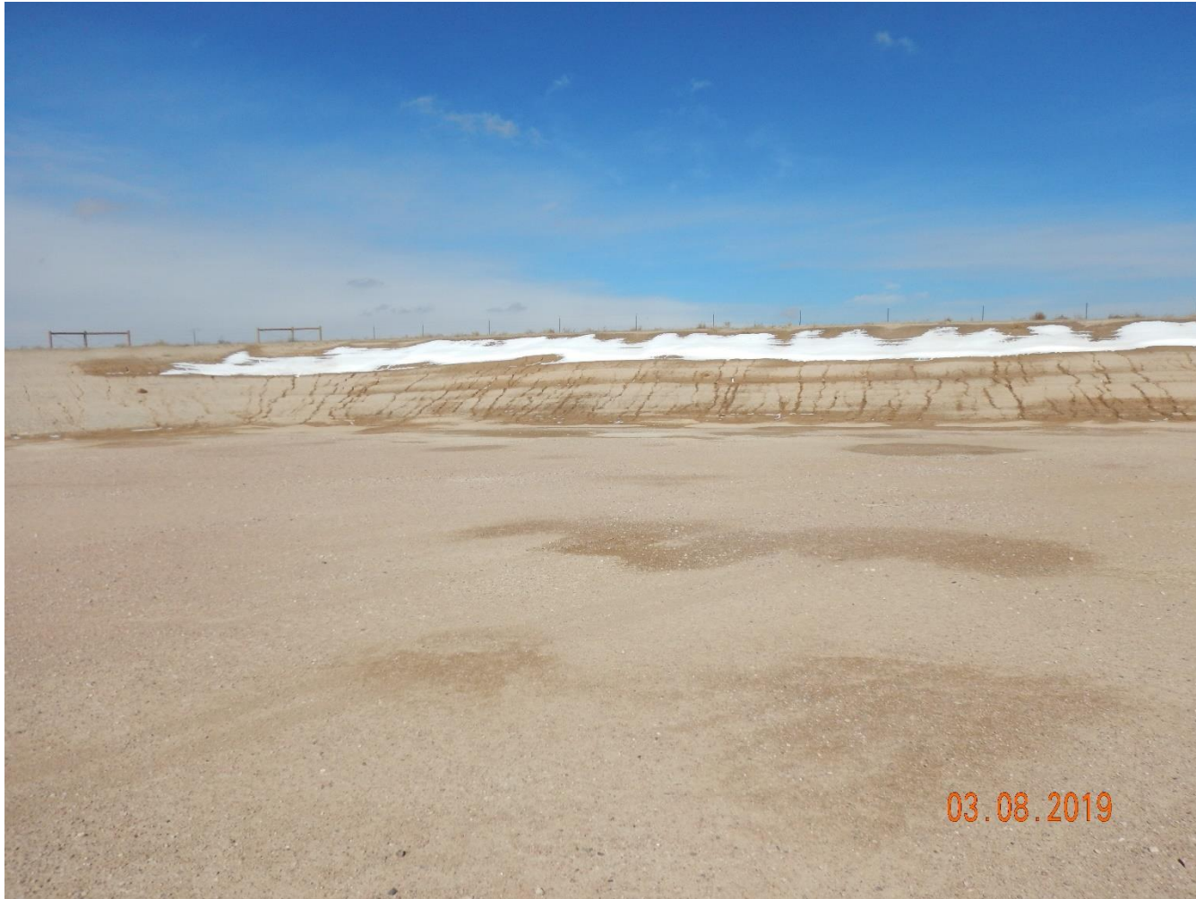
Photo 23: Photo taken from the northwest end of the pad, facing north. Photo shows stormwater erosion degradation on the slopes of the pad.
