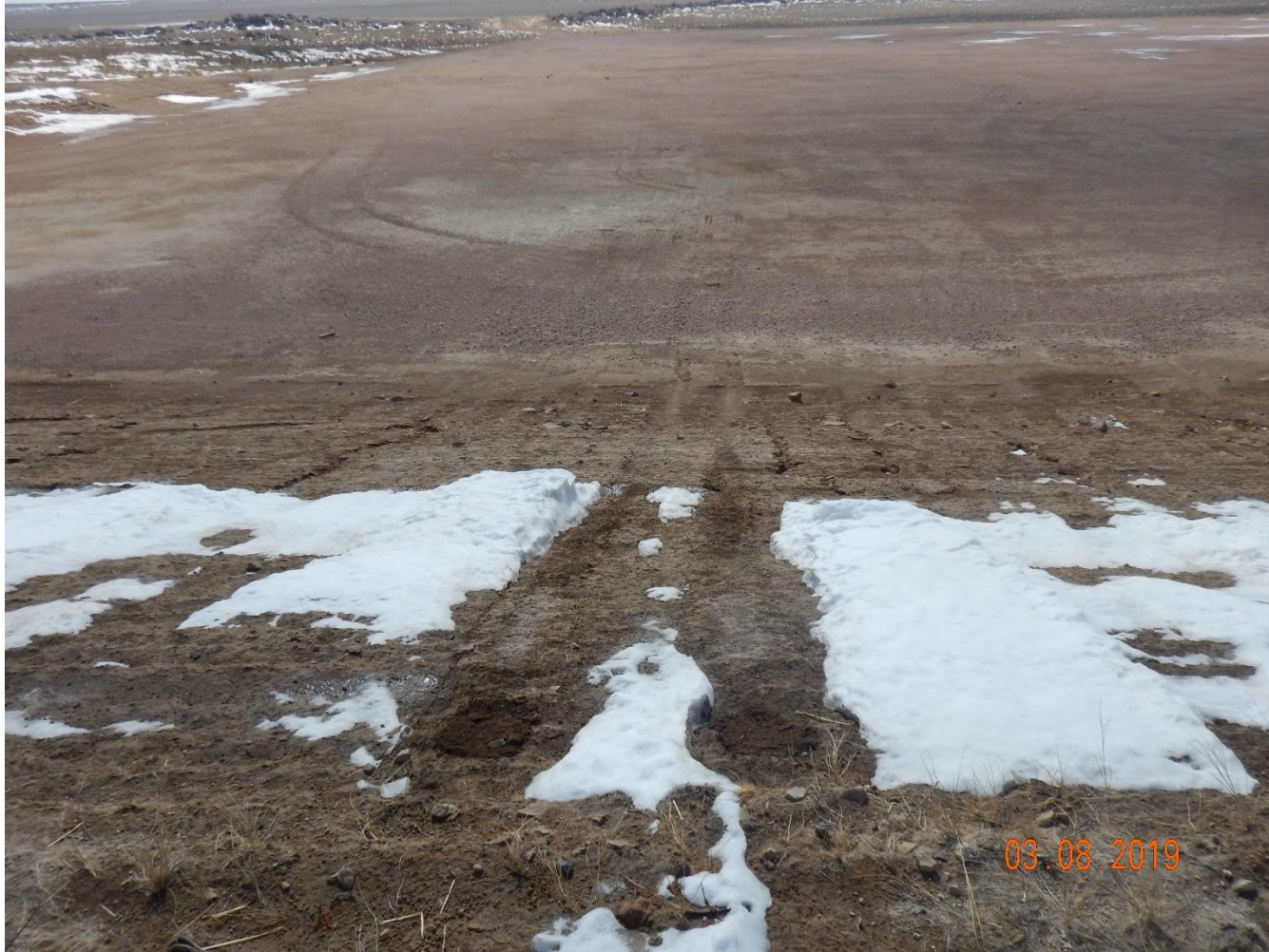
Photo 10: Photo taken from north end of the location, facing south. Photo shows tracks left by a vehicle that appears to have traveled upon the slopes and ditch of the location. This does not comply with surface disturbance minimization.
