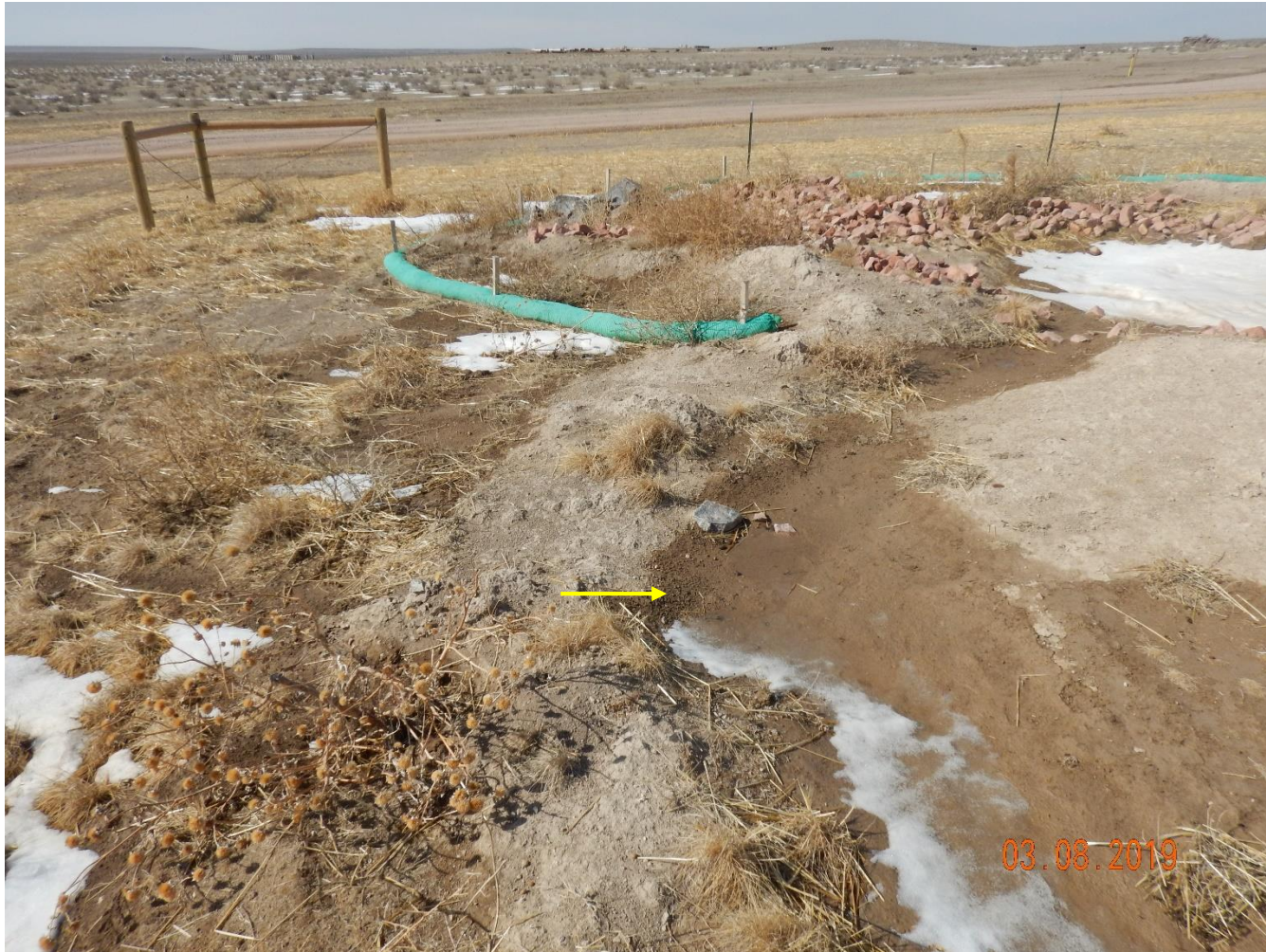
Photo 19: Photo taken from the sediment trap on the southwest corner of the pad. Photo shows areas of the ditch leading into the trap that has filled with sediment and is at equal elevation to the berm.
