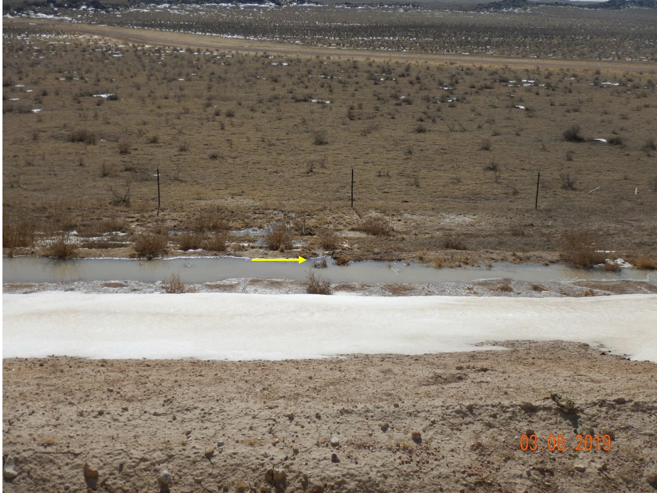
Photo 27: Photo taken from the south end of the pad, facing south. Photo shows section of the ditch that appears to have filled with sediment allowing stormwater to breach the BMP and discharge from location.
