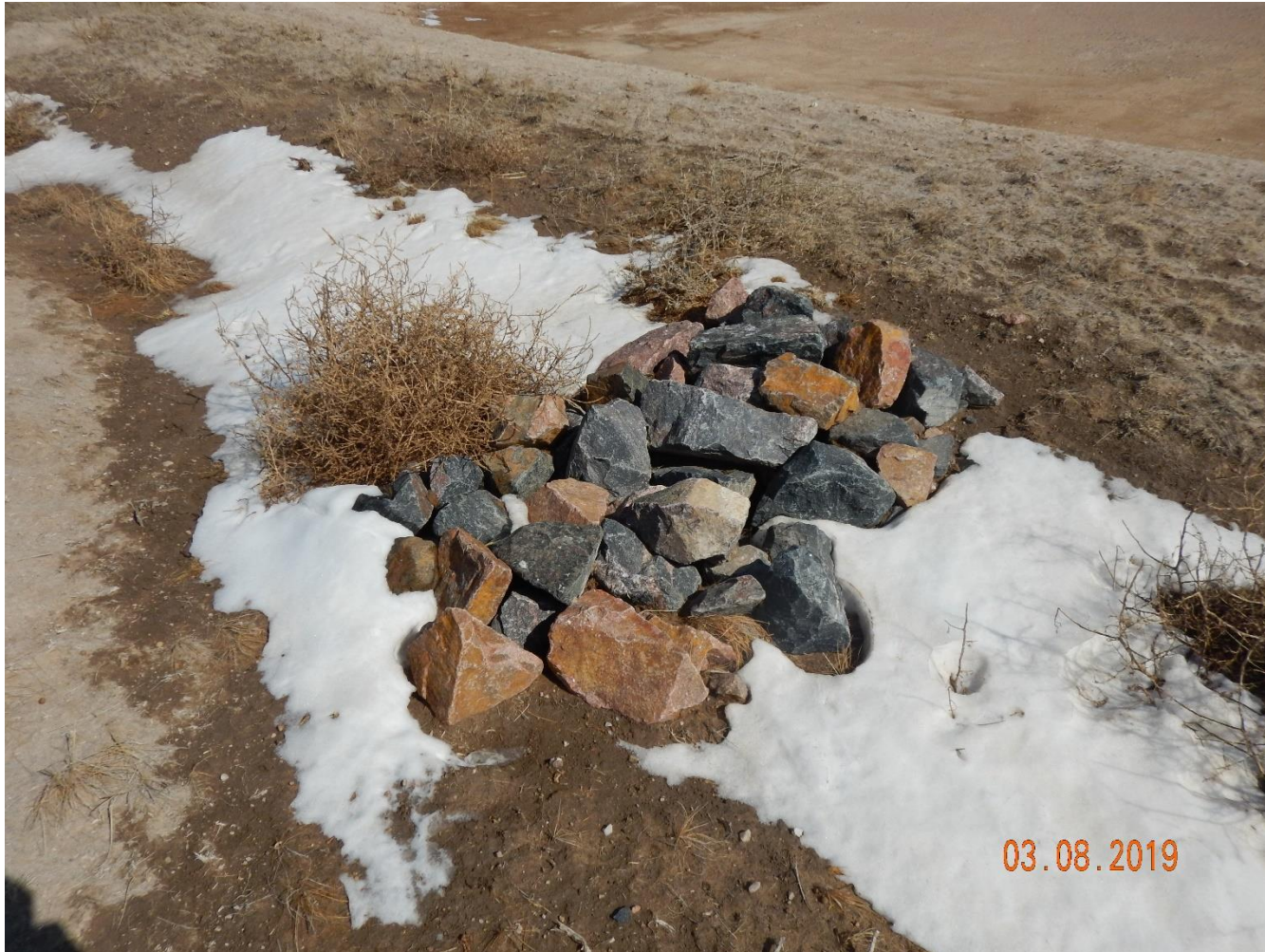
Photo 5: Photo taken from the stormwater ditch on the west end of the location. Photo shows velocity check. Operator appears to have only used large aggregate rock within check. This is not advised as stormwater will likely accelerate around the large rock and may contribute to erosion degradation within the ditch.
