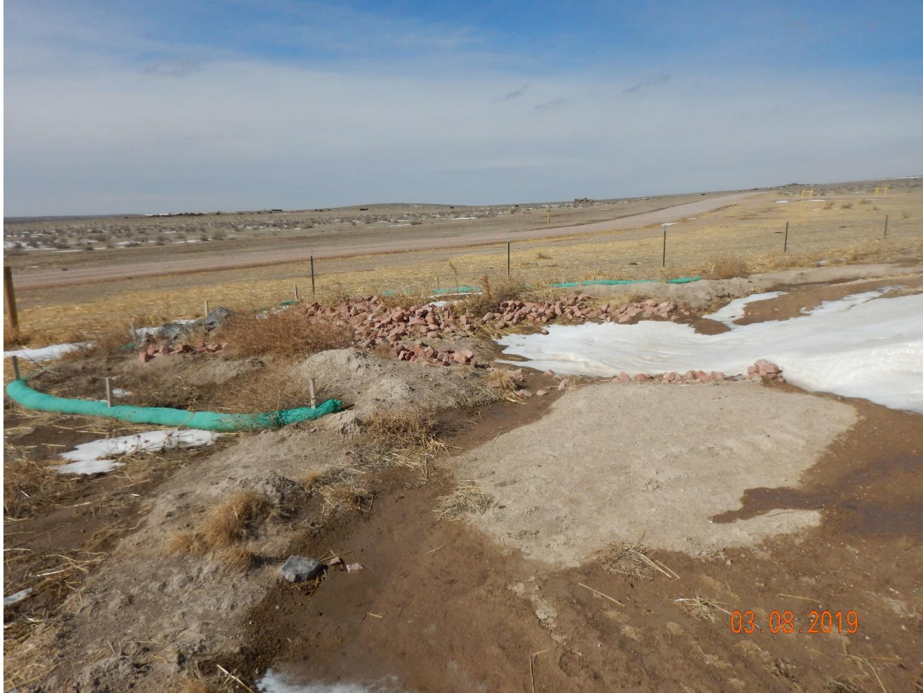
Photo 20: Photo taken from the sediment trap on the southwest corner of the pad, facing northwest. Sediment trap does not appear to be sufficient in size (length/width/depth) to mitigate stormwater run off from the pad.
