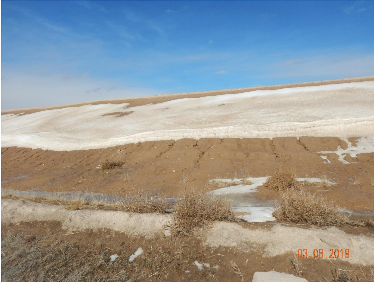
Photo 18: Photo taken from the south end of the location, facing north. Photo shows stormwater erosion degradation on the slopes of the pad.
