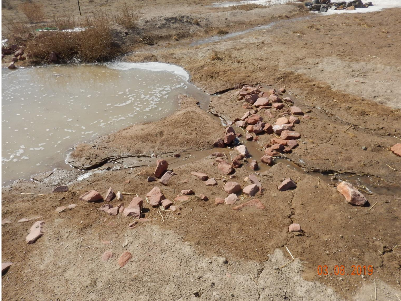
Photo 14: Photo taken from the sediment trap on the southeast corner of the location. Photo shows erosion degradation at the inlet of the BMP. Inlet protection appears to have either been “blown out” by stormwater discharge, or has become inundated with sediment and no longer in proper functioning condition.
