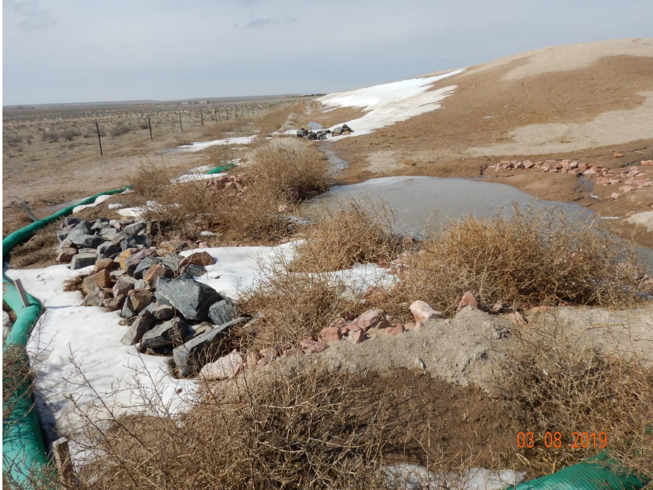
Photo 13: Photo of sediment trap on the southeast corner of the location.
