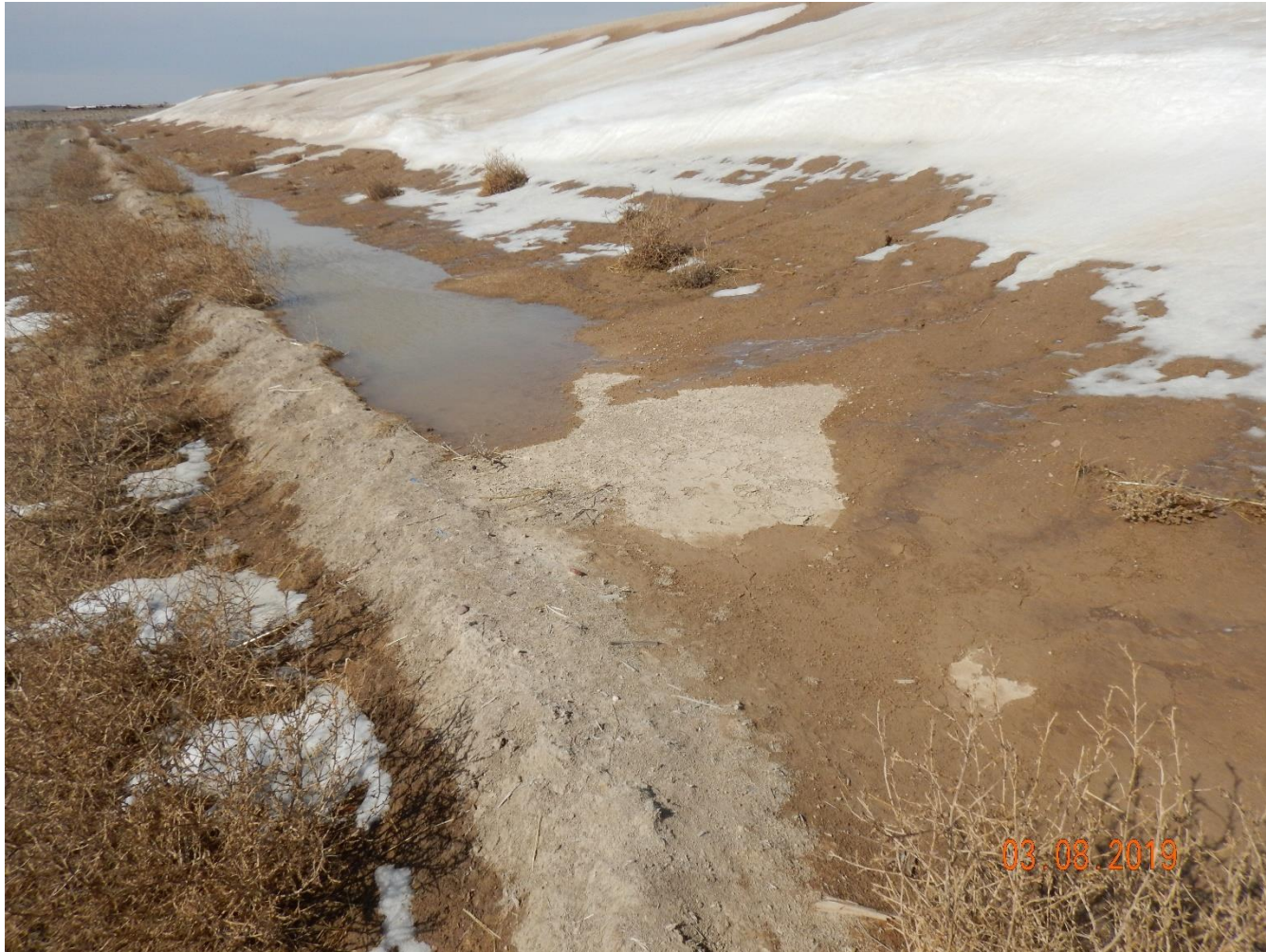
Photo 16: Photo taken from the stormwater ditch on the south end of the location, facing northwest. Photo shows ditch has filled with sediment. Maintenance required.
