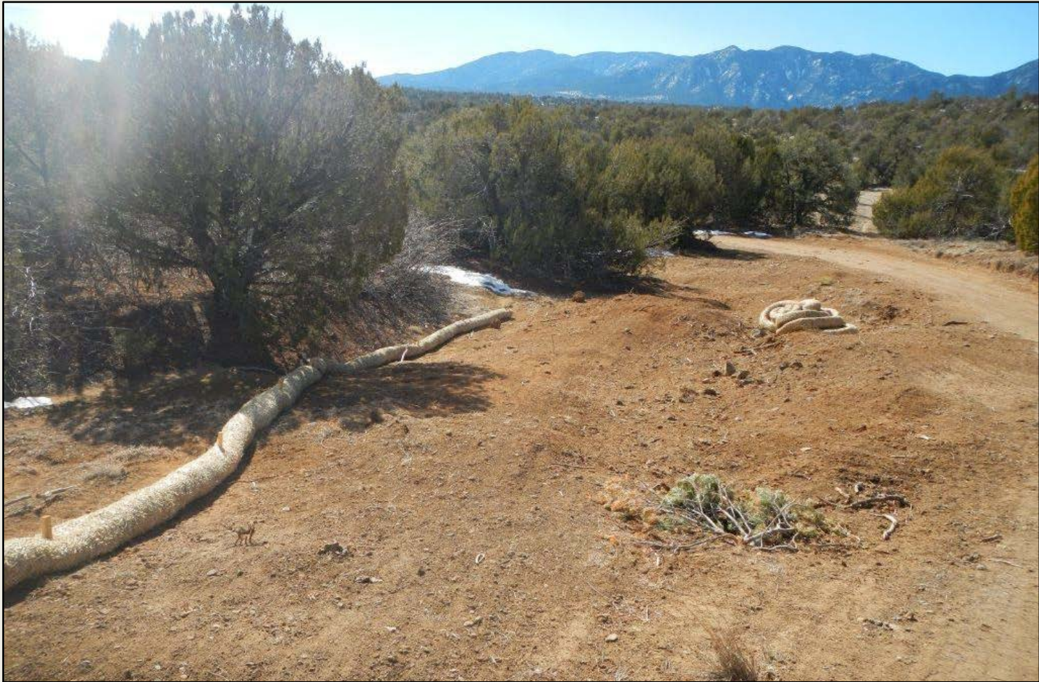
Photo 6. View of area near the access entrance where wattle installation is not completed.
