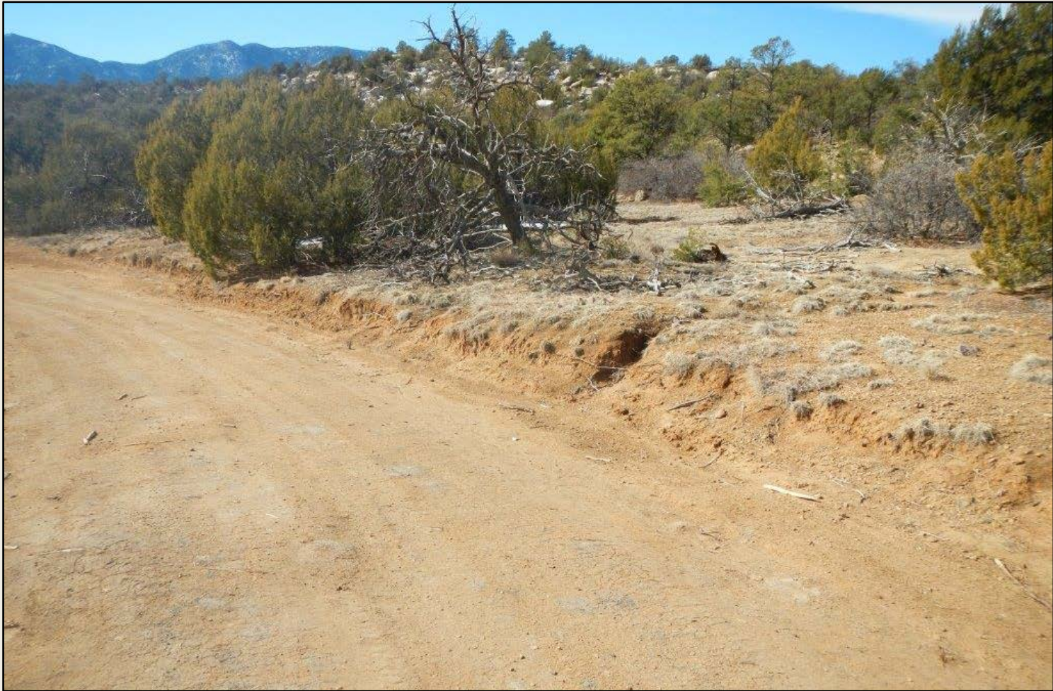
Photo 7. View of area along access where run-on controls and stabilization are needed. Additional areas along access where stormwater needs to be managed and controlled remain.
