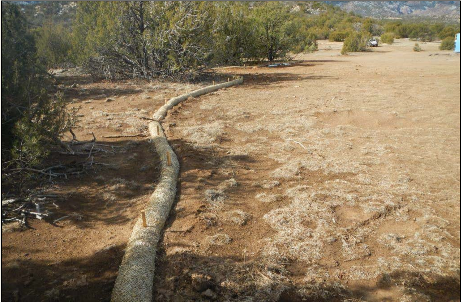
Photo 2. View of the eastern project area from the eastern corner facing southward. Wattles are placed around the perimeter of the project area.
