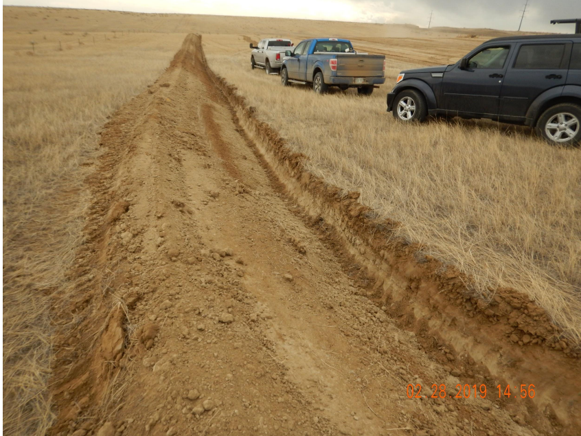
Photo 3. Photo taken from the northeastern perimeter of location, facing South. Photo illustrates a ditch and berm BMP installed around the Location. Operator shall stabilize the berm BMP, as an unconsolidated berm BMP is not a proper functioning BMP. Operator indicated that the berm would be stabilized the day of this inspection.
