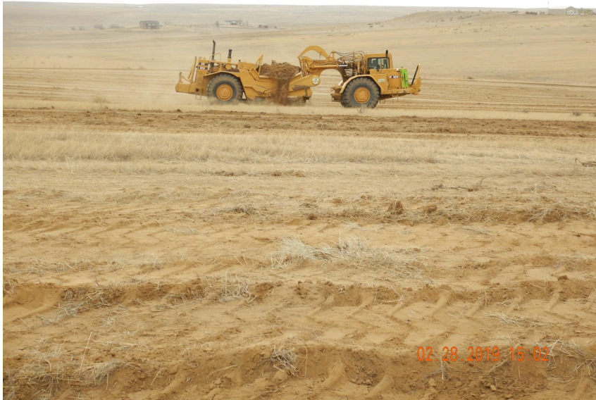
Photo 5. Photo taken from the western perimeter of the location, facing East. Photo illustrates Operator in-process of salvaging topsoil.
