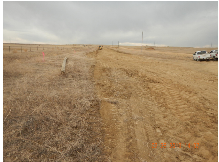
Photo 2. Photo taken from the entrance of location, facing West. Photo illustrates access road in-process of being constructed. Operator salvaged and stored topsoil from the access.
