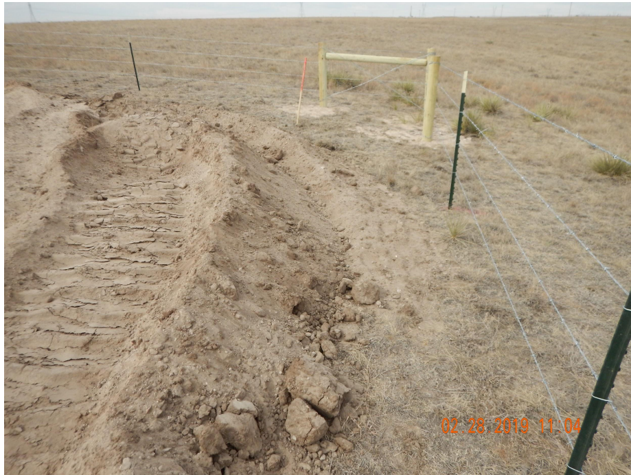
Photo 7. Photo taken from the northwestern perimeter of location, facing West. Photo illustrates unconsolidated soil material without a perimeter BMP. Operator on Location stated that wattle BMPs would be installed around the remainder of the location.
