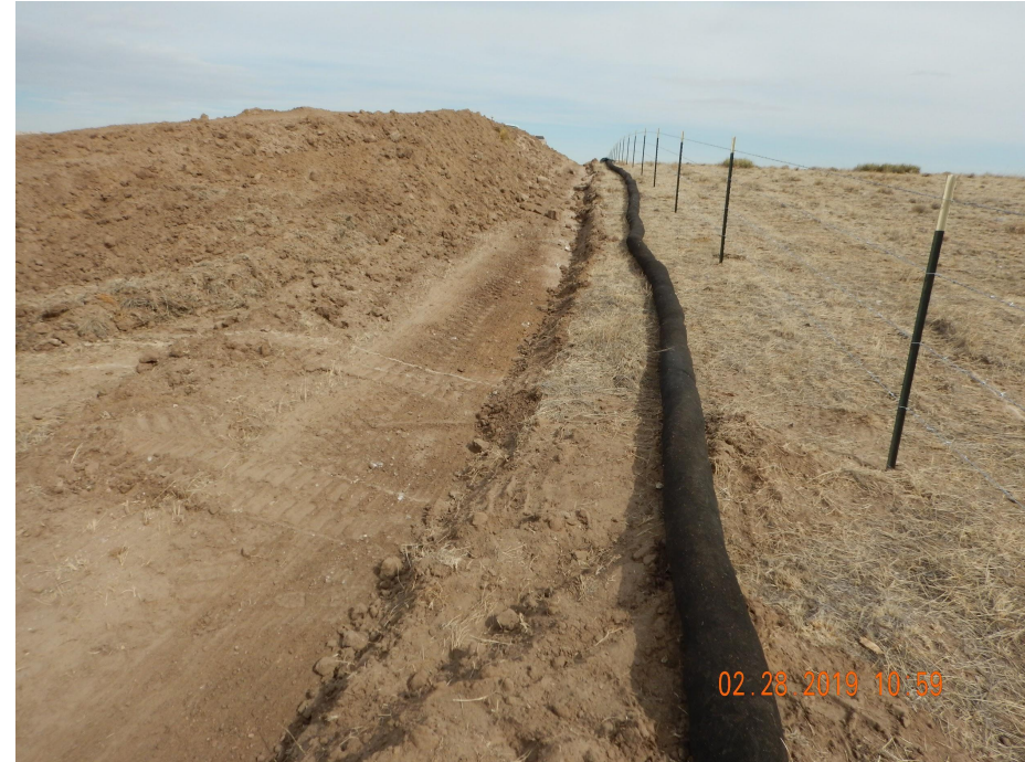
Photo 4. Photo taken from the southeastern perimeter of location, facing North. Photo illustrates the topsoil stockpile and perimeter BMPs. Wattle BMP has not been staked.
