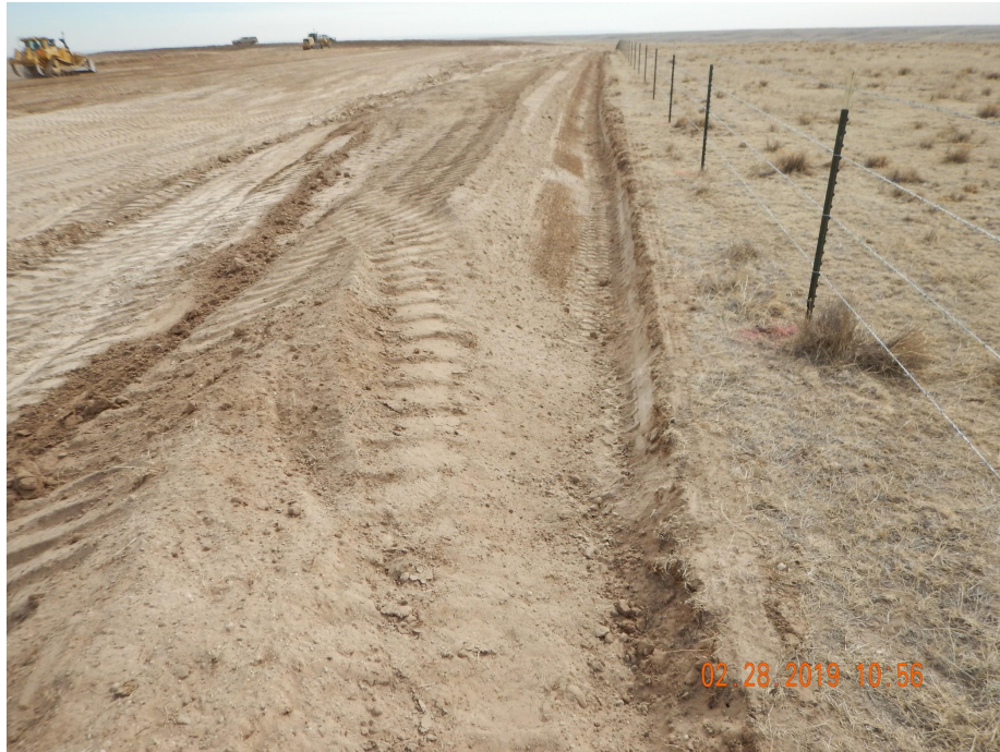
Photo 1. Photo taken from the southwestern perimeter of location, facing East. Photo illustrates a berm and ditch BMP. Operator shall stabilize the berm BMP, as unconsolidated soil material is susceptible to wind and water erosion.
