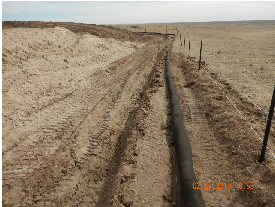
Photo 3. Photo taken from the southeastern perimeter of location, facing East. Photo illustrates wattle BMP which has not been staked. Wattle BMP should be installed to the outermost disturbance area.
