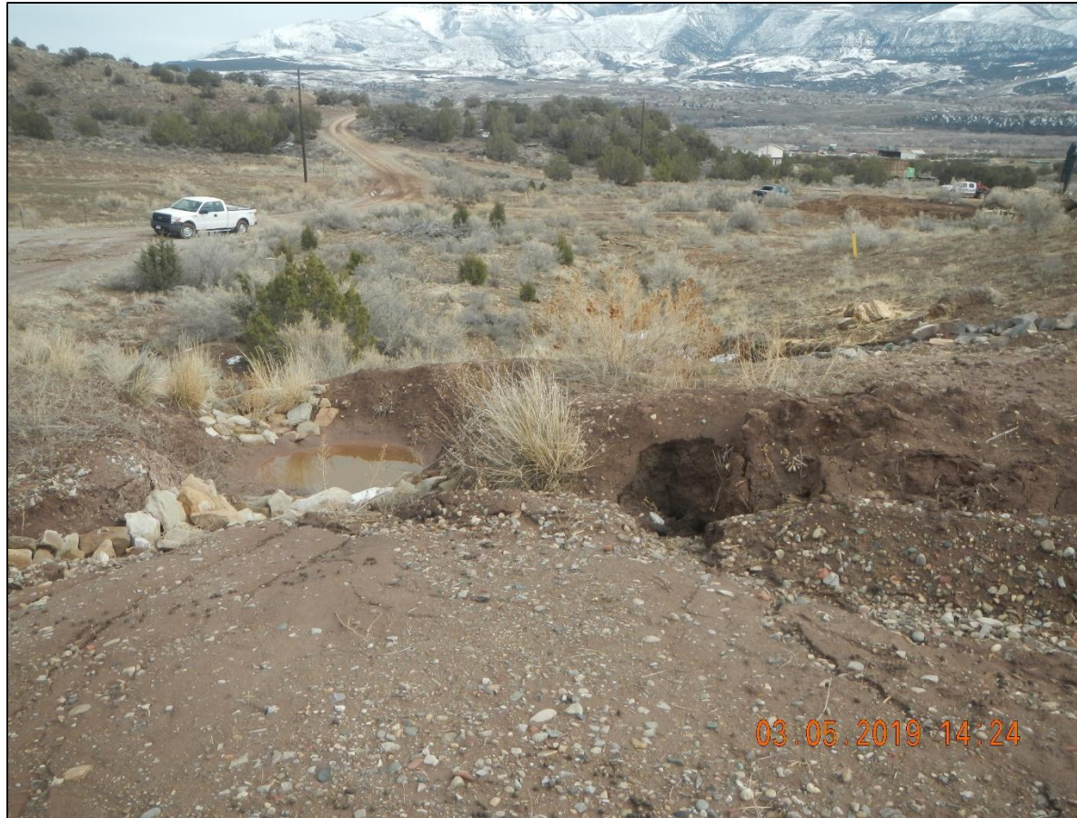
Washout of ditch wall at checkdam.
