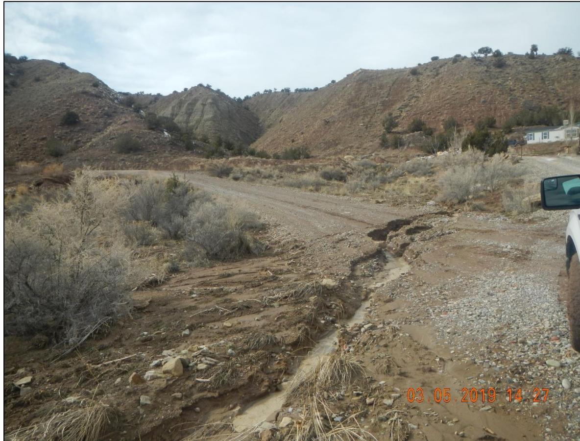
Washout on access road into location.
