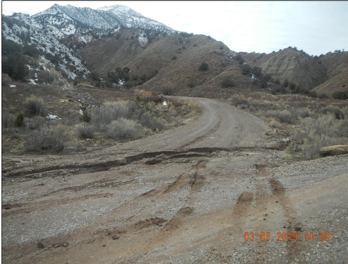
Washout on access road into location.
