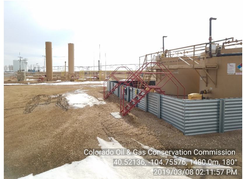
Photo #2 UPV 3-1G6 Former Battery site Now belongs to SRC Energy
