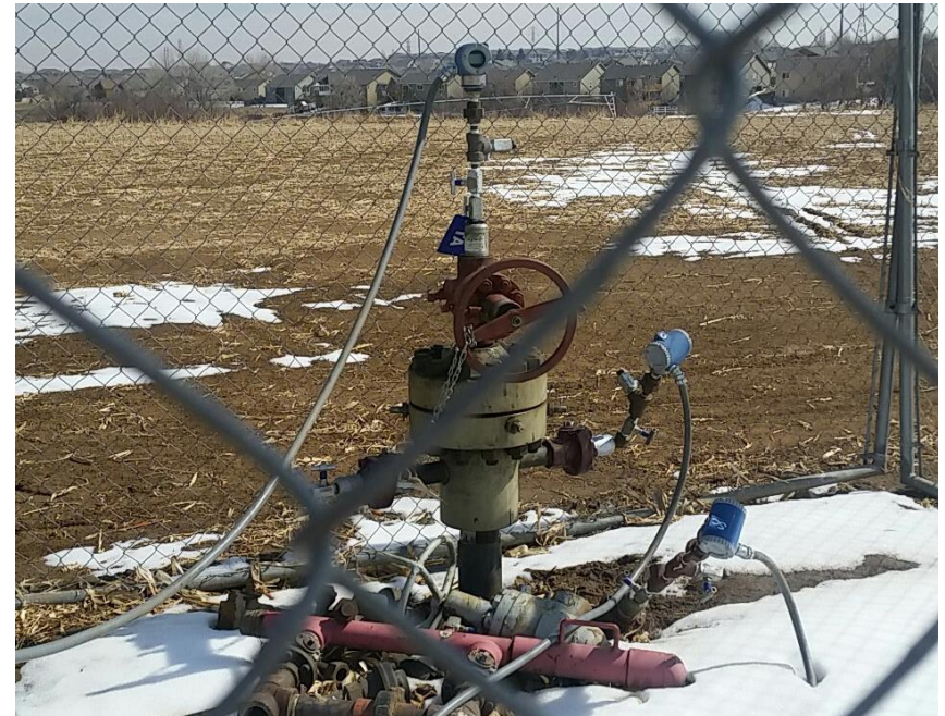
Photo 2 – Wellhead TA well
