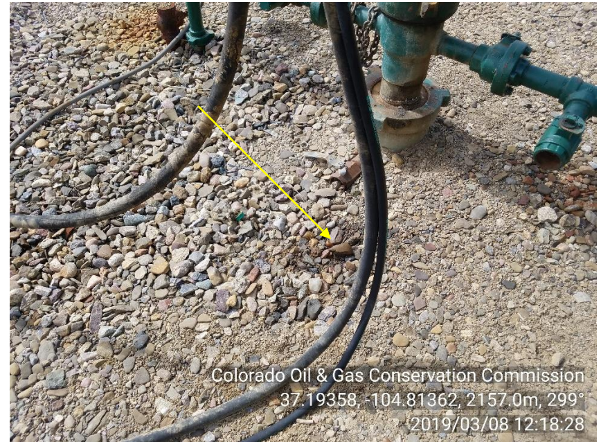
PHOTO 4: IMPACTED SOIL BENEATH 1" HYDRAULIC LINE.
