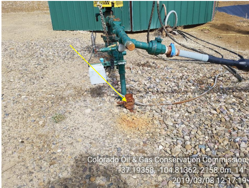
PHOTO 7: UNMARKED UNUSED RISER. VALVE IS BROKE
