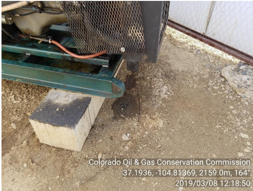
PHOTO 5: APPEARS ENGINE IS LEAKING OIL. IMPACTED SOIL BENEATH FRONT OF ENGINE SKID.
