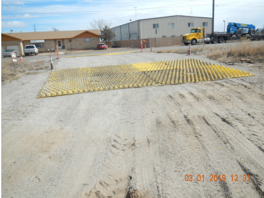
Photo 7. Photo taken from the access road off CR 27, facing East. Appears Operator has installed tracking pads and gravel to potentially limit tracking onto the county road.
