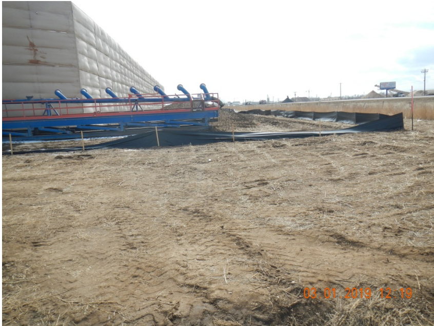
Photo 1. Photo taken from the northwestern perimeter of the location, facing South. Photo illustrates the installed silt fence BMP is not in proper functioning condition.
