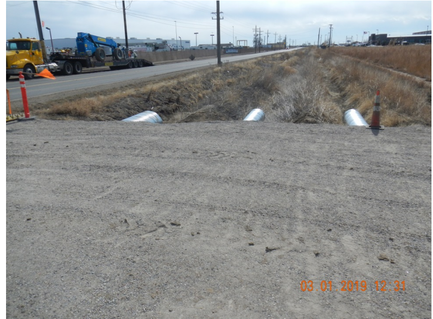
Photo 8. Photo taken from the access road off CR 27, facing South. Photo depicts the three new culverts installed.
