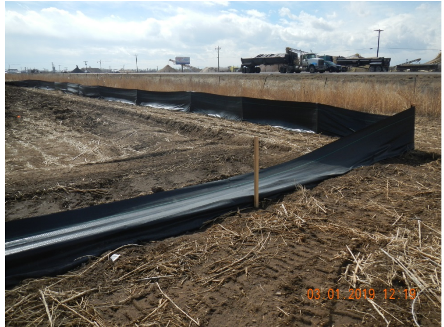
Photo 2. Photo taken from the northwestern perimeter of the location, facing Southeast. See comments from Photo 1. There is also a ditch and berm BMP installed around the perimeter. However there are no sediment traps with stabilized outlets observed on location at the time of inspection.
