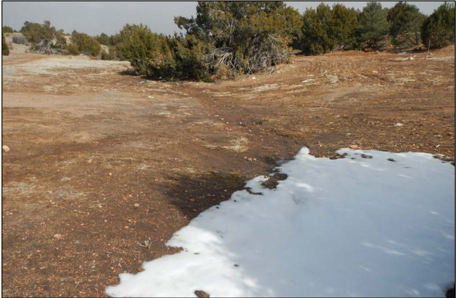
Photo 5. View of swale in the northern project area where snow melt is causing erosion. Stormwater controls are needed to stabilize erosion and sediment run-off from the project area.
