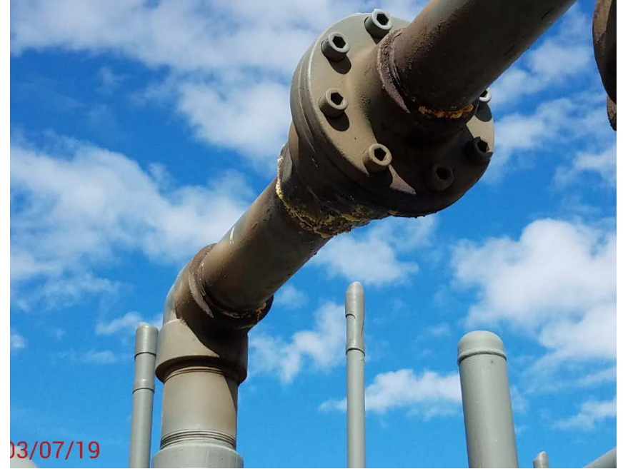
Location Photo #6, Leaking flow line on top of vessel.
