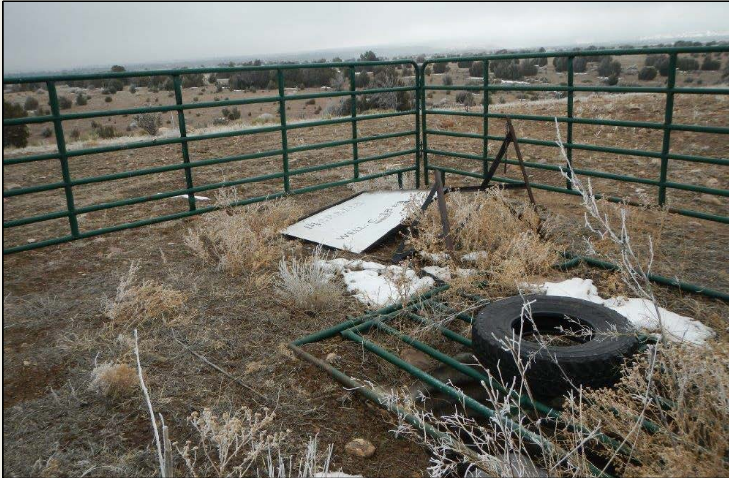
Photo 3. View of debris around well head area. Well cellar should be properly closed to prevent wildlife entrapment.
