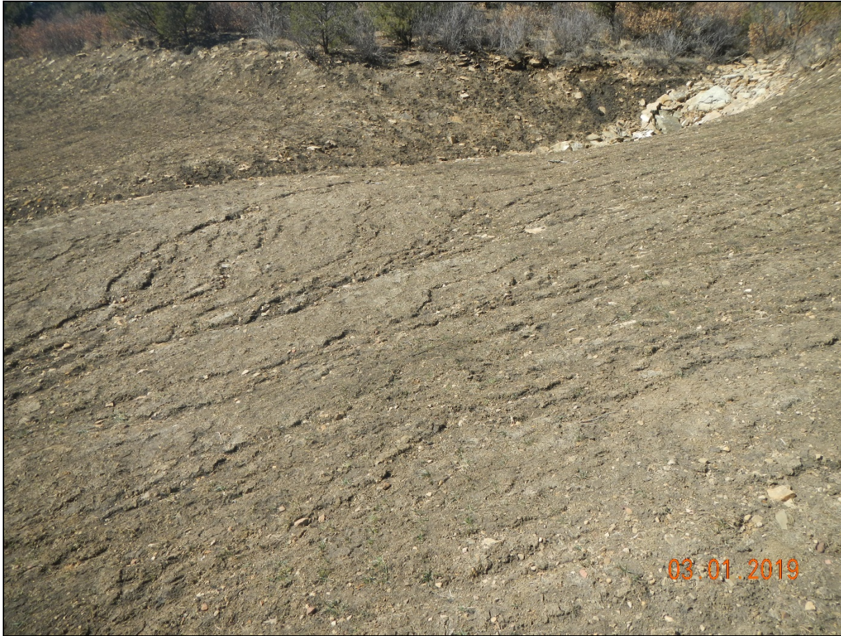
Photo 2. There is little vegetation establishing at the beginning of the reclaimed road. This area may require additional seeding.
