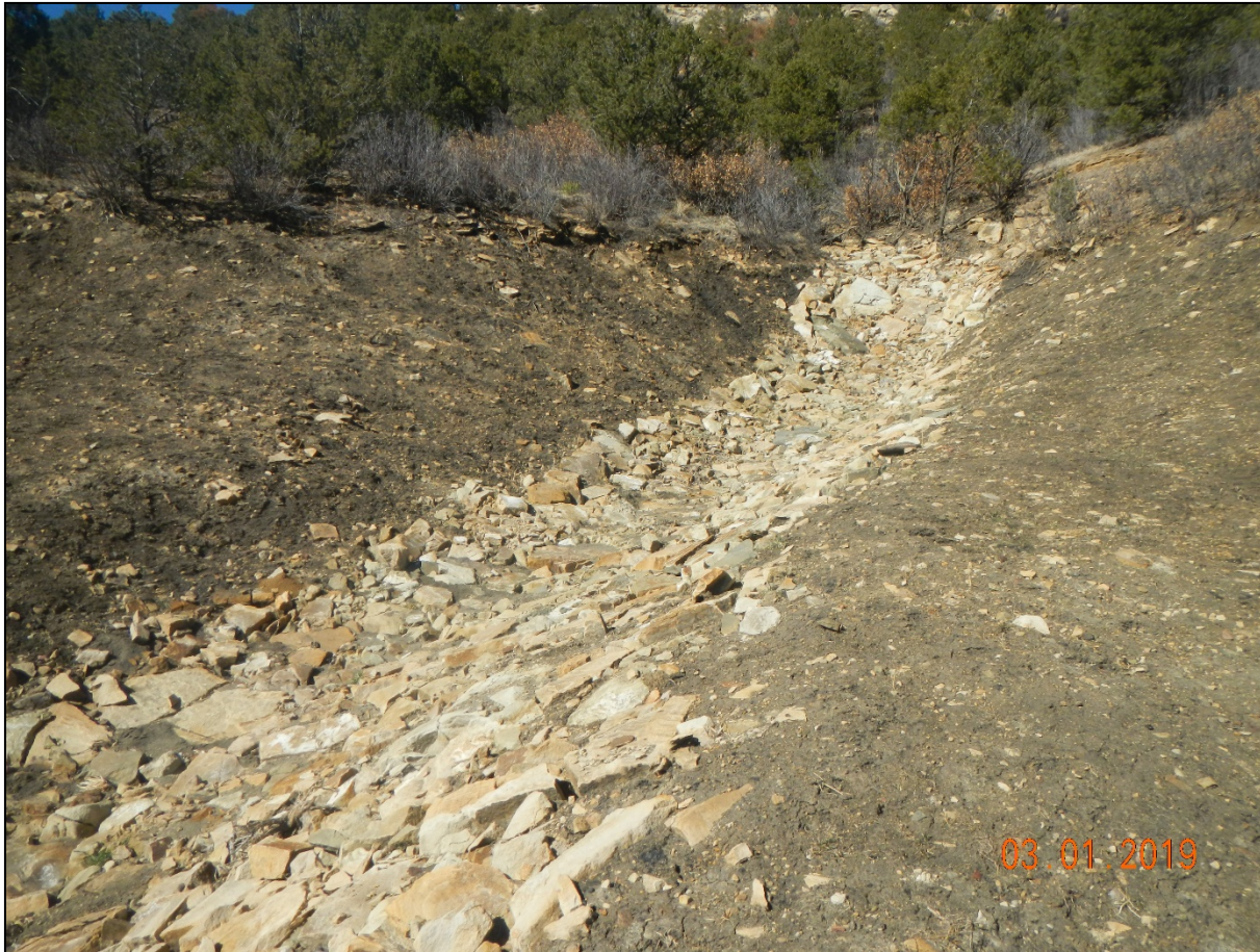
Photo 3. Rock rip/rap is placed in the drainage channel.
