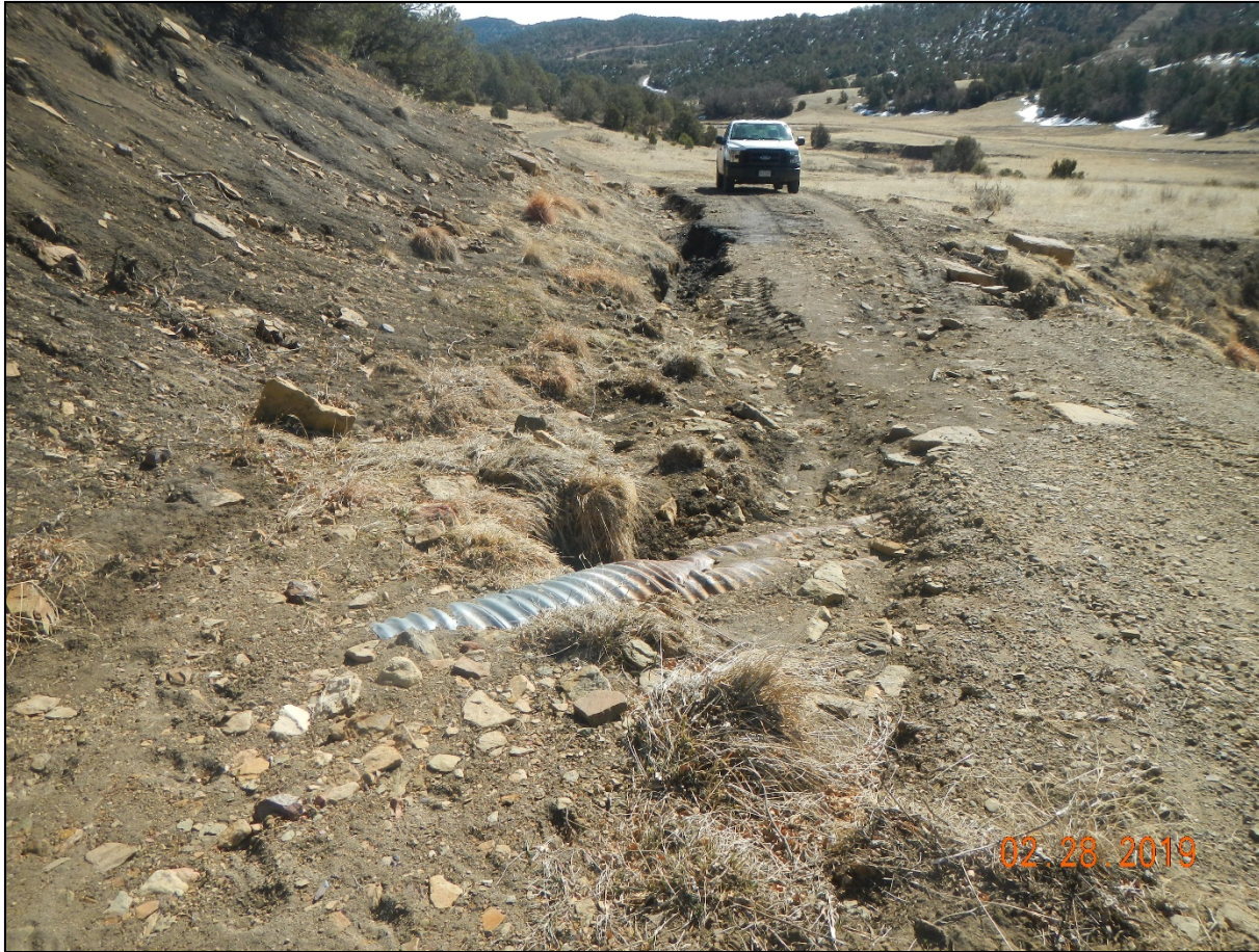
Photo 3. Facing southwest at Lat/Long:37.09966,-104.73441. The culvert is filled in with sediment and erosion is occurring down the road.
