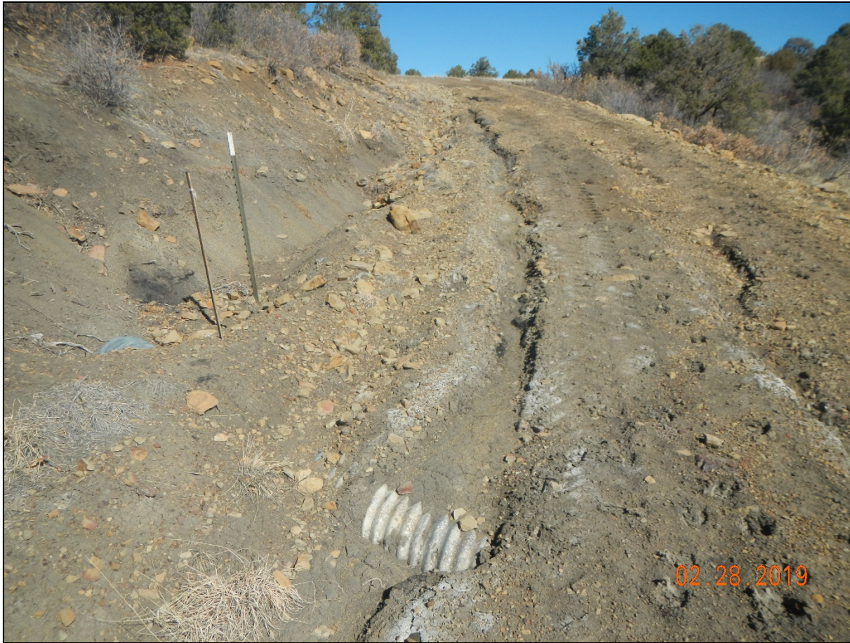
Photo 4. Further along the road traveling toward the top of the ridge near the TAD POLE #21-12 location. Erosion is occurring down the road past the culvert.
