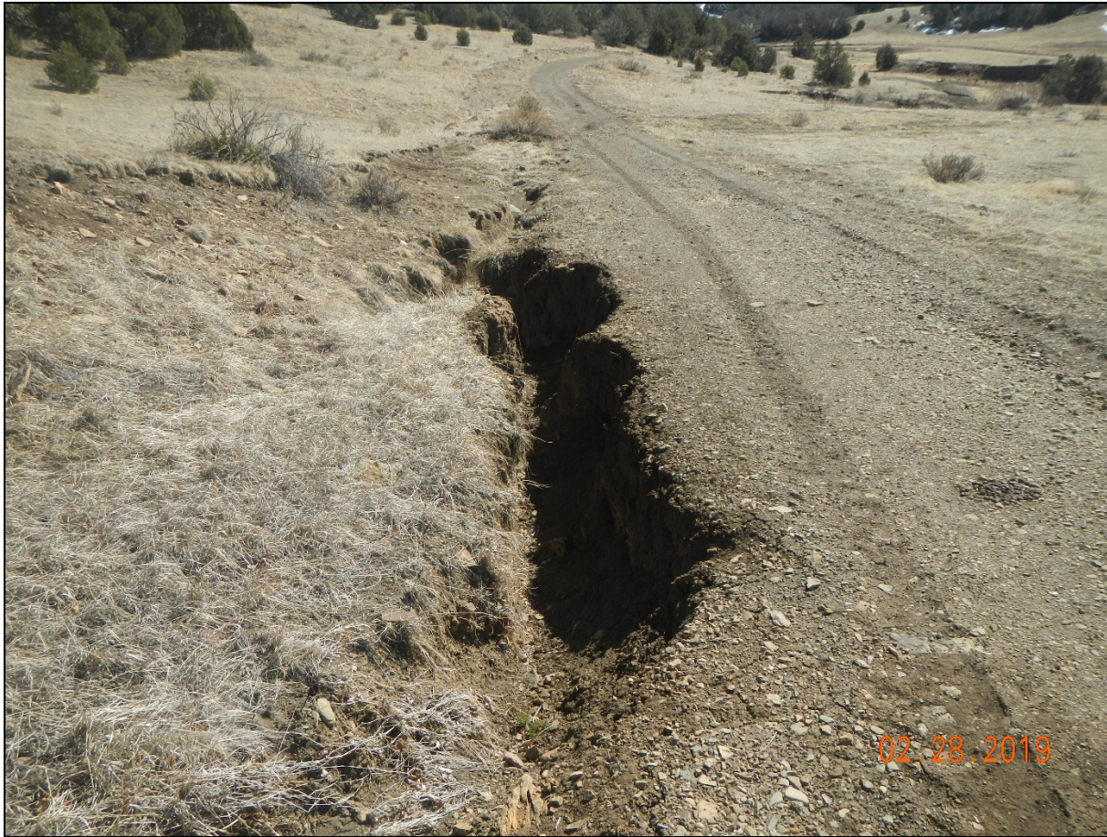
Photo 2. Erosion is occurring along the access road. Facing southeast.
