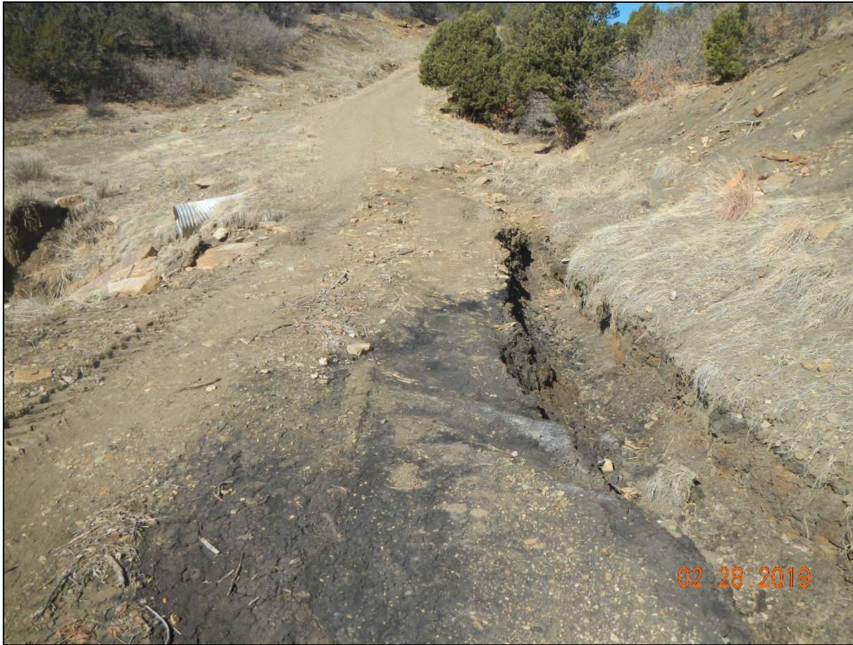
Photo 1. Erosion is occurring along the access road at Lat/Long:37.09966,-104.73441. Facing northwest.
