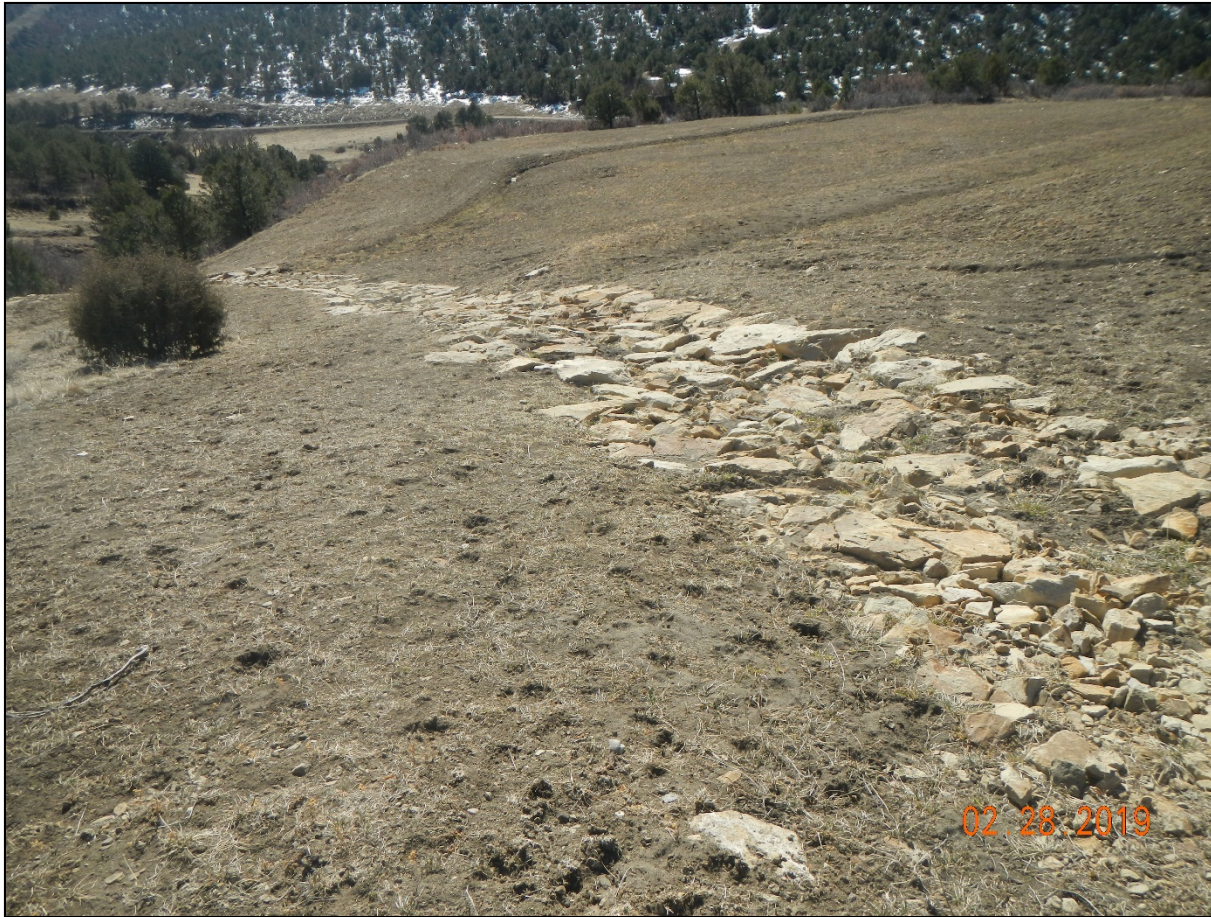
Photo 2. Rock rip/rap is placed in the drainage channel.
