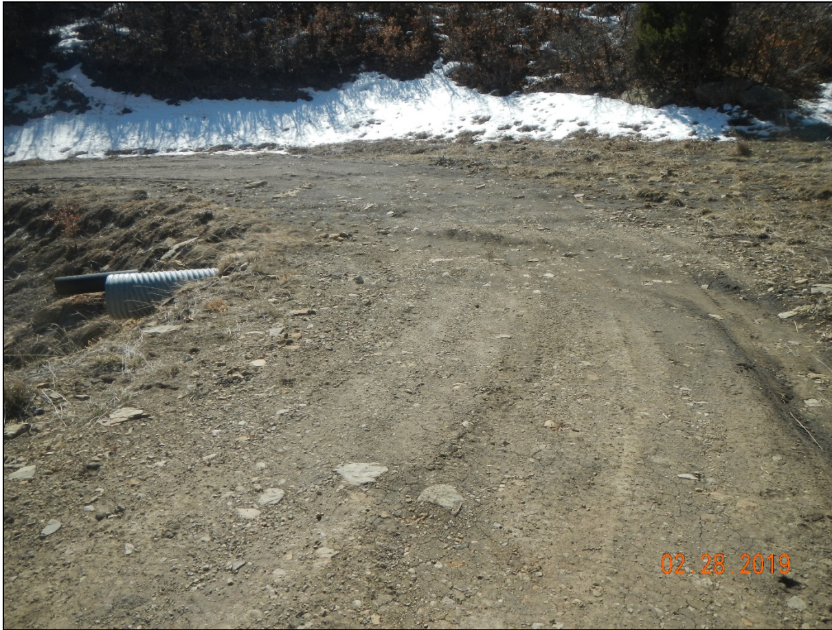
Photo 8. Culvert is filled in with sediment and stormwater is flowing across the road. Lat/Long:37.09338,-104.74751
