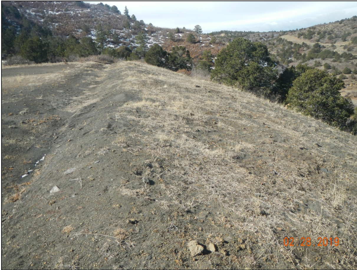
Photo 7. Facing toward the south side of the location. Vegetation is established along the fill slope.
