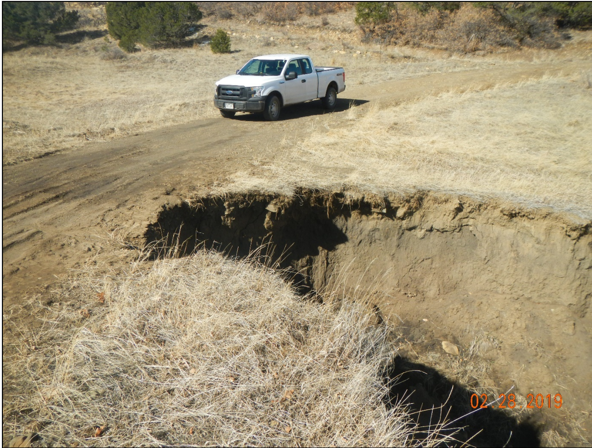
Photo 4. Erosion is cutting into the road, approximately 8-10 ft. deep.
