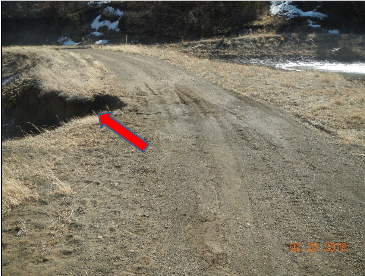
Photo 1. Erosion is occurring along the access road at Lat/Long:37.08649,-104.75026.
