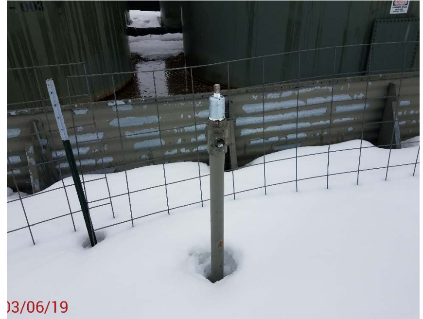
Location Photo #8, unused/unmarked flow line riser by tank battery.
