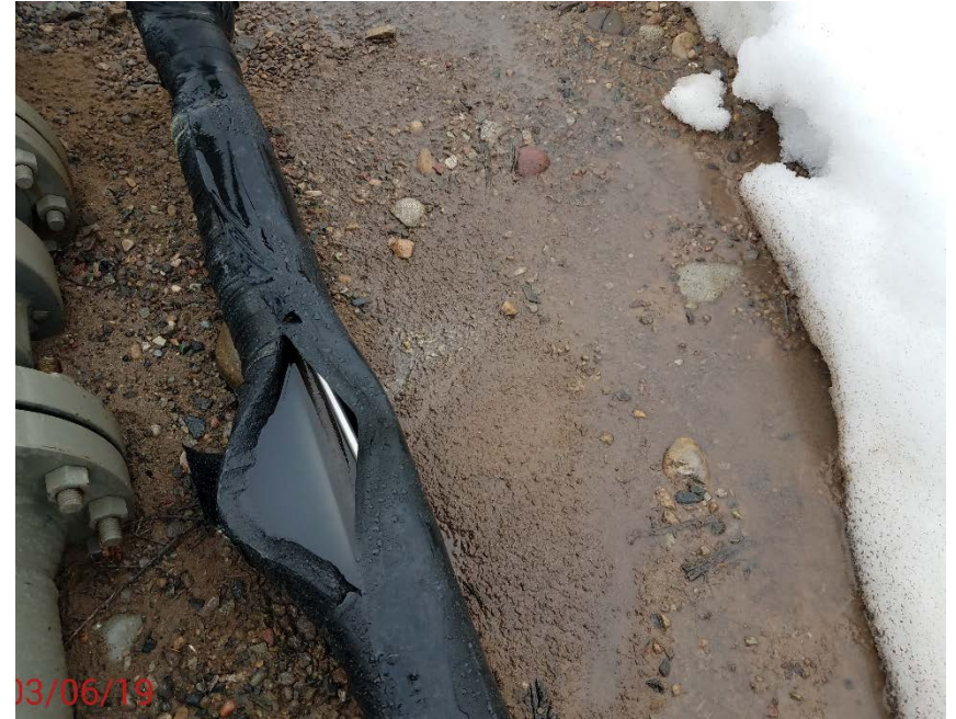
Location Photo #14, Area of the leak.
