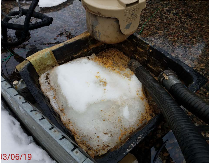
Location Photo #7, condensate in secondary drip pan.
