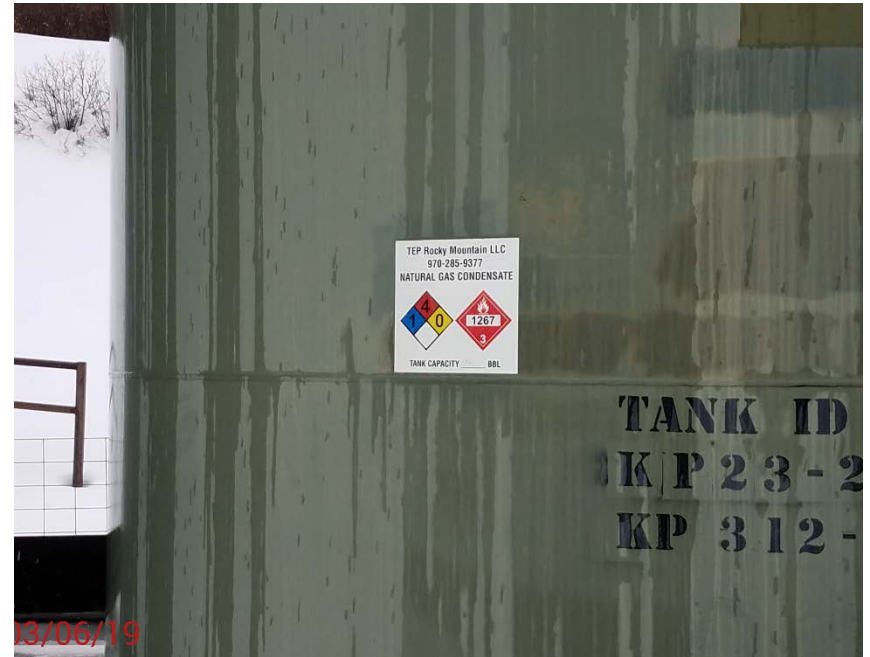
Location Photo #6, Missing BBL quantity on 4 production tanks.
