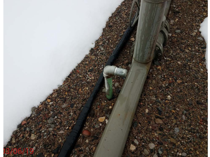
Location Photo #4, Unused/unmarked flowline riser, near separators.
