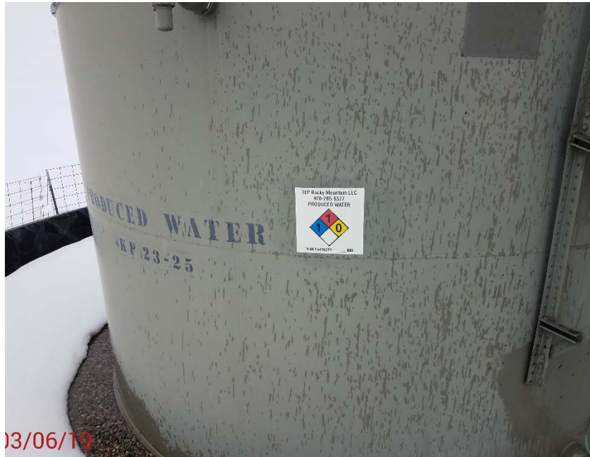
Location Photo #5, Missing BBL quantity on 4 production tanks.
