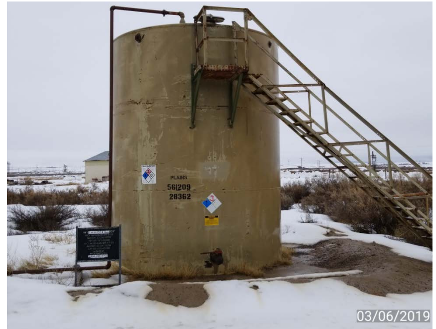
Photo 2. Tank battery.
