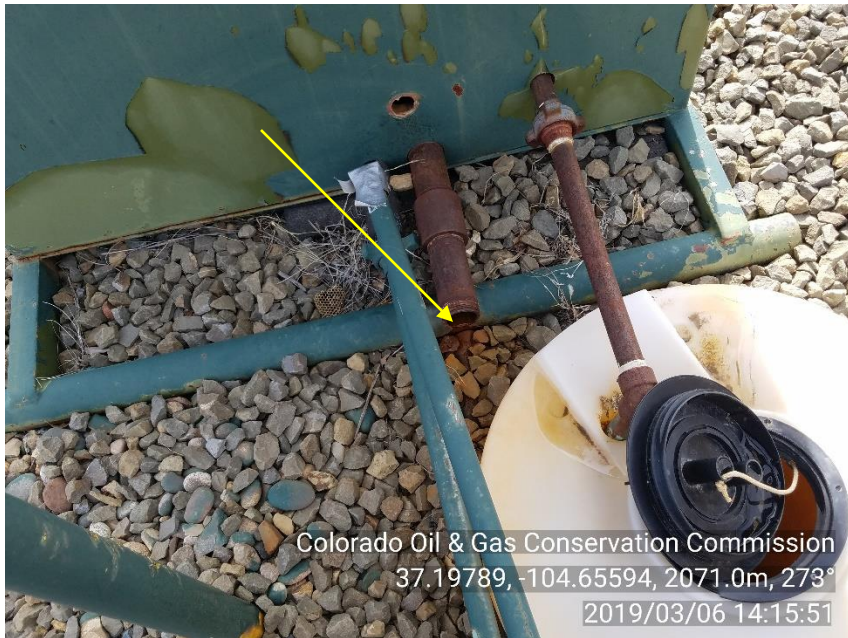
PHOTO 3: PRODUCED WATER DRIPPING FROM SEPARATOR TO THE GROUND
