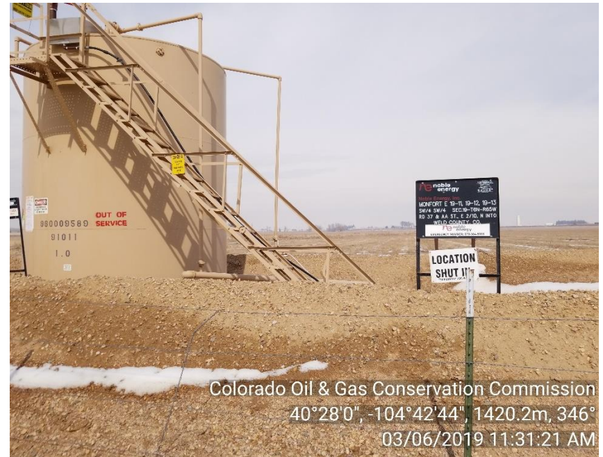
Photo 2: Centralized Tank Battery
