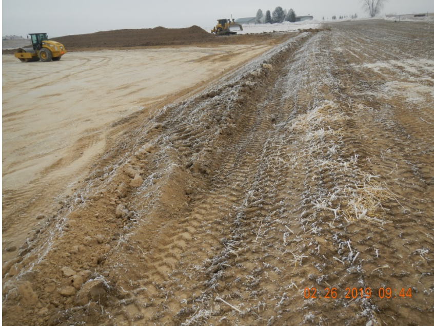
Photo 1. Photo taken from the northwestern perimeter of the location, facing South. Photo illustrates a compacted BMP that has been installed around the perimeter of the location.
