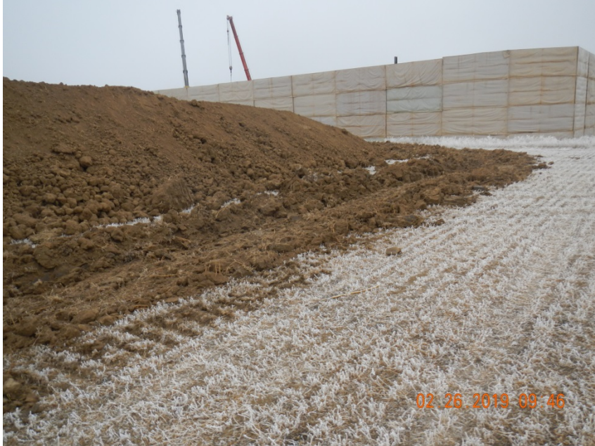
Photo 5. Photo taken from the southern perimeter of the location, facing East. Photo illustrates the topsoil stockpile being stored along the southern area is not stabilized . See comments from Photo 4.
