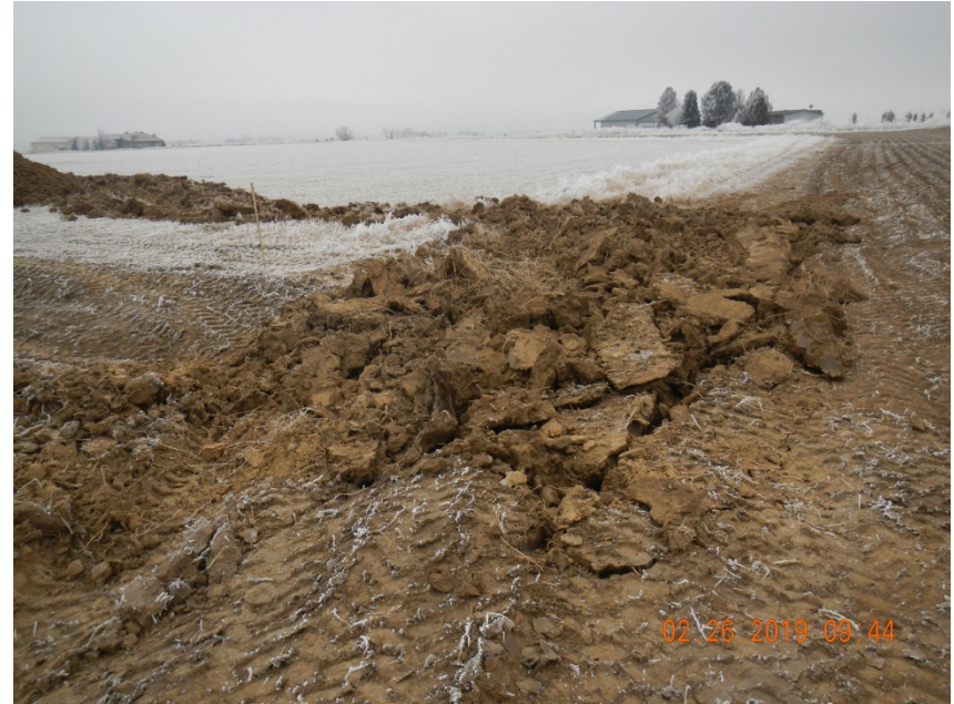
Photo 4. Photo taken from the southwestern perimeter of the location, facing South. A ditch and berm BMP was being installed around the topsoil pile at the time of the inspection and have not been completed due to lack of compaction and has not been installed with best engineering practices. However this should have been complete at the time of inspection because major dirt work activities had already been completed.
