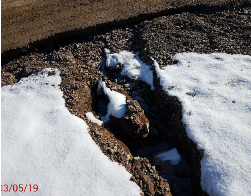
Location Photo #9, Access road is washed out.
