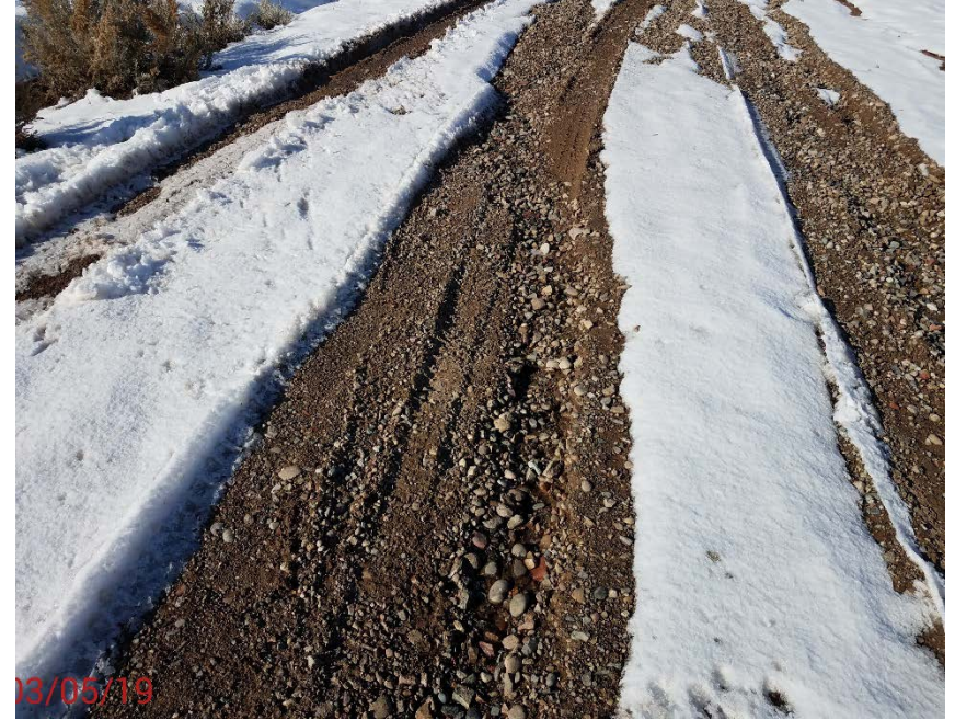
Location Photo #10, Rilling on the access road.
