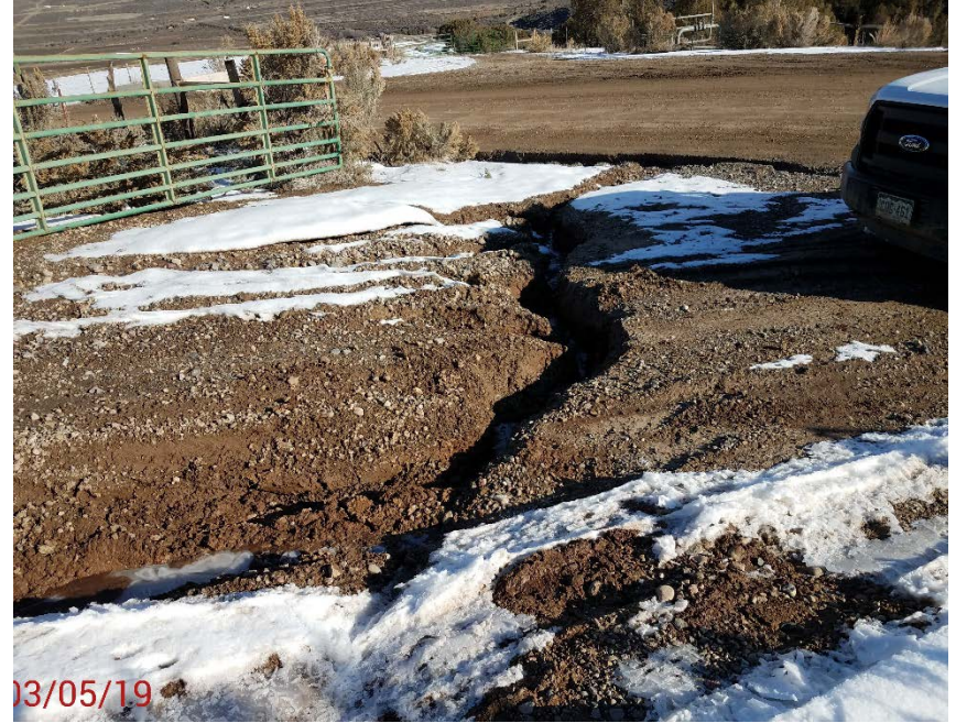
Location Photo #6, Access road is washed out.
