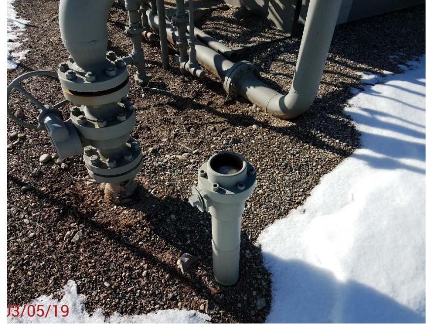
Location Photo #4, Unused/unmarked flow line near Separators.
