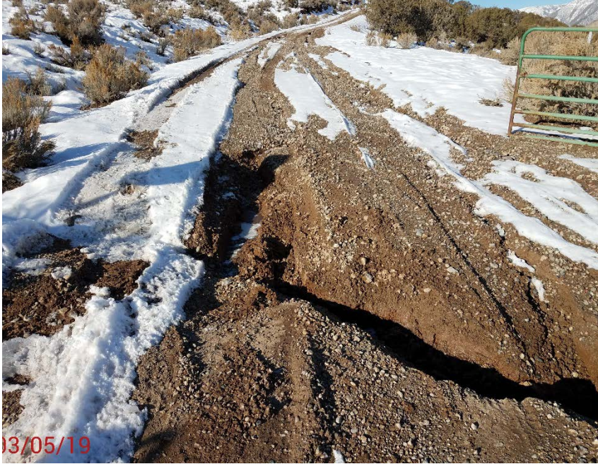
Location Photo #5, Access road is washed out.
