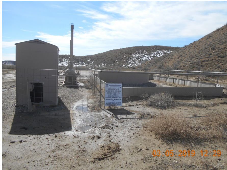
Meter housing and Separator Tank battery. Metal berms and fencing
