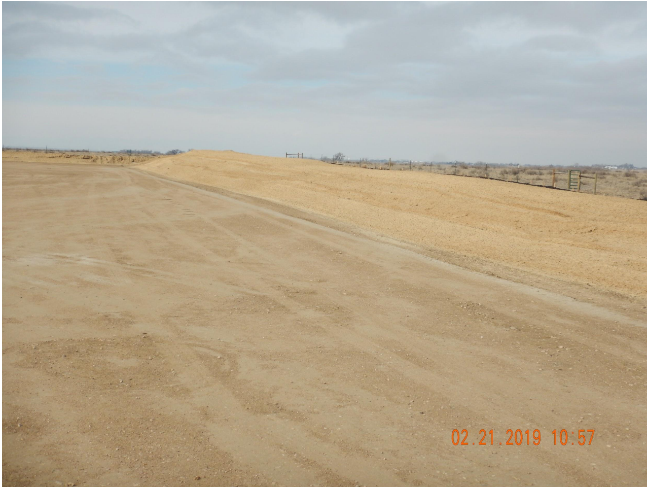
Photo 1. Photo taken from the northern well pad, facing West. Photo illustrates the topsoil stockpile that has been temporarily stabilized with hydromulch. In addition, Operator shall ensure topsoil is protected from weed establishment.
