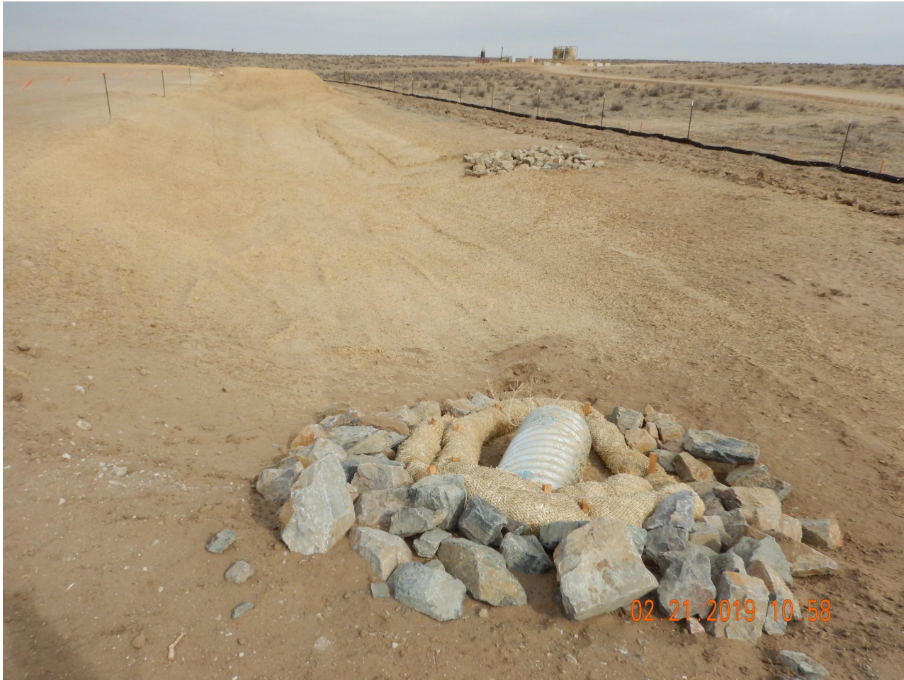
Photo 5. Photo taken from the southeastern well pad, facing North. Photo illustrates a retention area with a stabilized outlet. Hydromulch has also been applied within the retention area.
