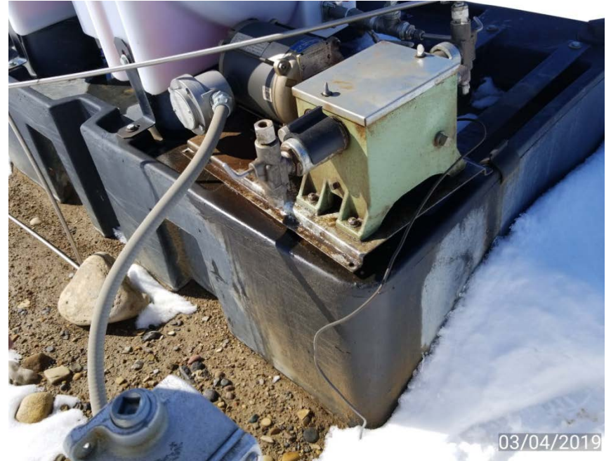
Photo 2. Inhibitor pump leaking fluid outside of secondary containment.
