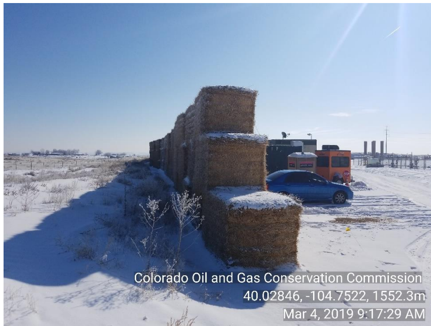
Photo 3 Loc pic Staw bails for sound walls
