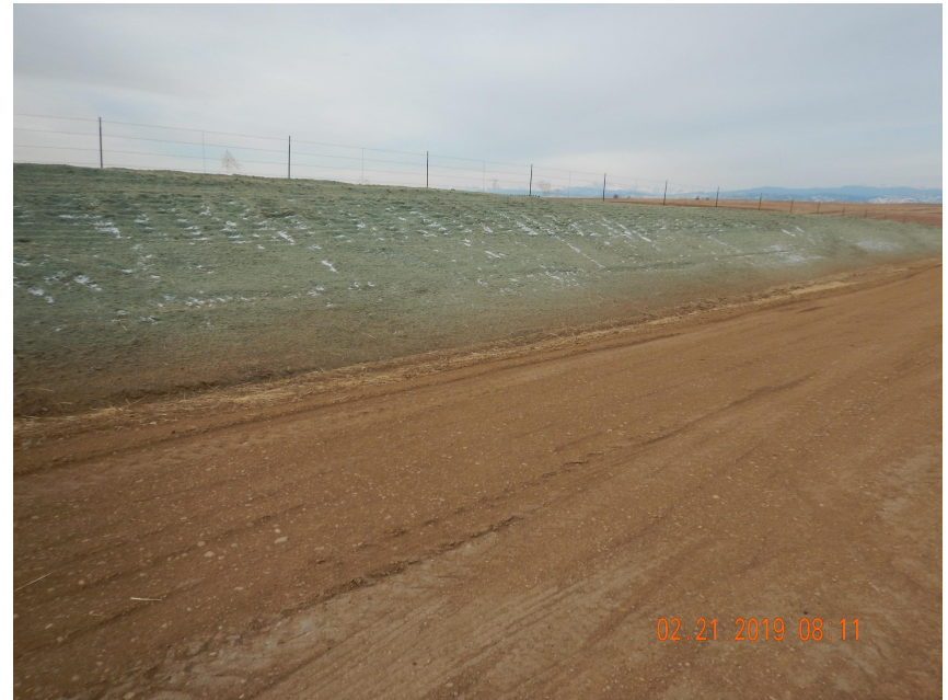
Photo 2. Photo taken from the southern location, facing West. Photo illustrates the cut slope has been temporarily stabilized with equipment tracking and hydromulch.
