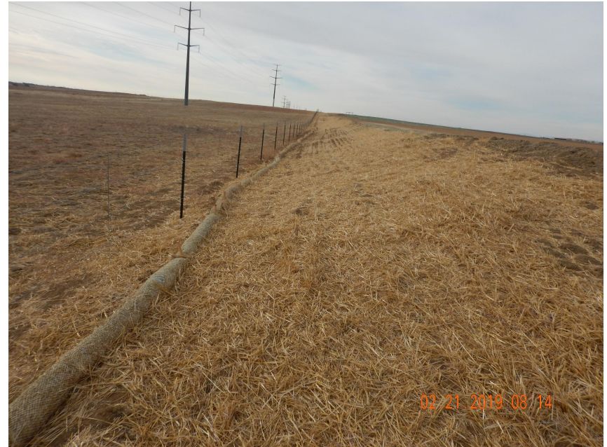
Photo 6. Photo taken from the northeastern perimeter of location, facing South. Photo illustrates the Operator performed the previous corrective action to properly install the straw wattle BMP.
