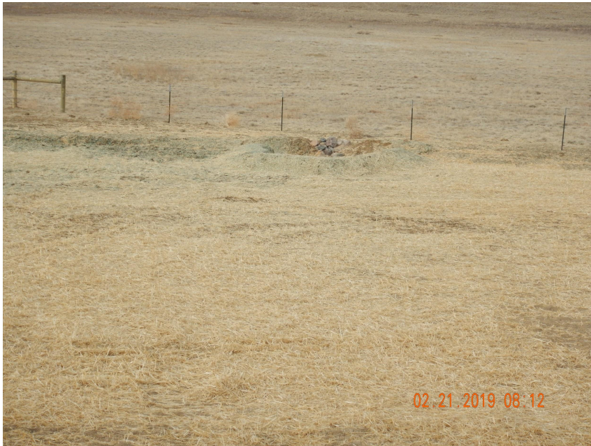
Photo 3. Photo taken from the southwestern perimeter of the location, facing West. Photo illustrates the western fill slope area has been seeded and straw crimped with mulch. The sediment trap is only for any runoff from the western fill slope area which includes the topsoil stockpile.
