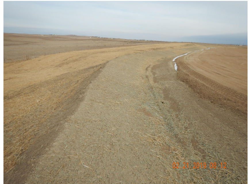
Photo 4. Photo taken from the southwestern well pad, facing North. Photo illustrates the ditch and berm has been temporarily stabilized with hydromulch. Also, photo illustrates the topsoil stockpile has been temporarily stabilized with equipment tracking, seeded and straw crimped with mulch.
