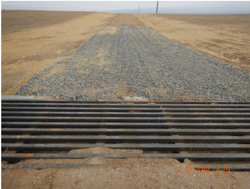
Photo 1. Photo taken from the entrance of location, facing North. Photo illustrates a tracking device BMP that appears to be in proper function condition and the outer perimeter of the access road has seeded and straw crimped with mulch.
