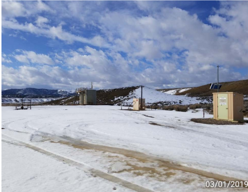
Photo 1. Location looking southwest.
