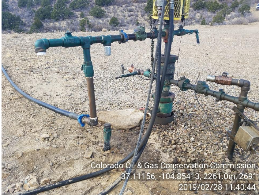
PHOTO 3: DISCHARGE LINE BYPASSING SEPARATOR/ IMPACTED SOIL NEAR WELLHEAD.
