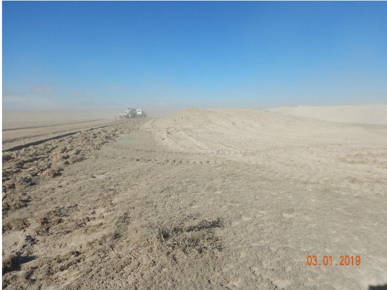
Photo 8: Photo taken from the southeast end of the location, facing west. Photo shows ongoing wind erosion degradation transporting sediment off of the location and soil stockpiles.
