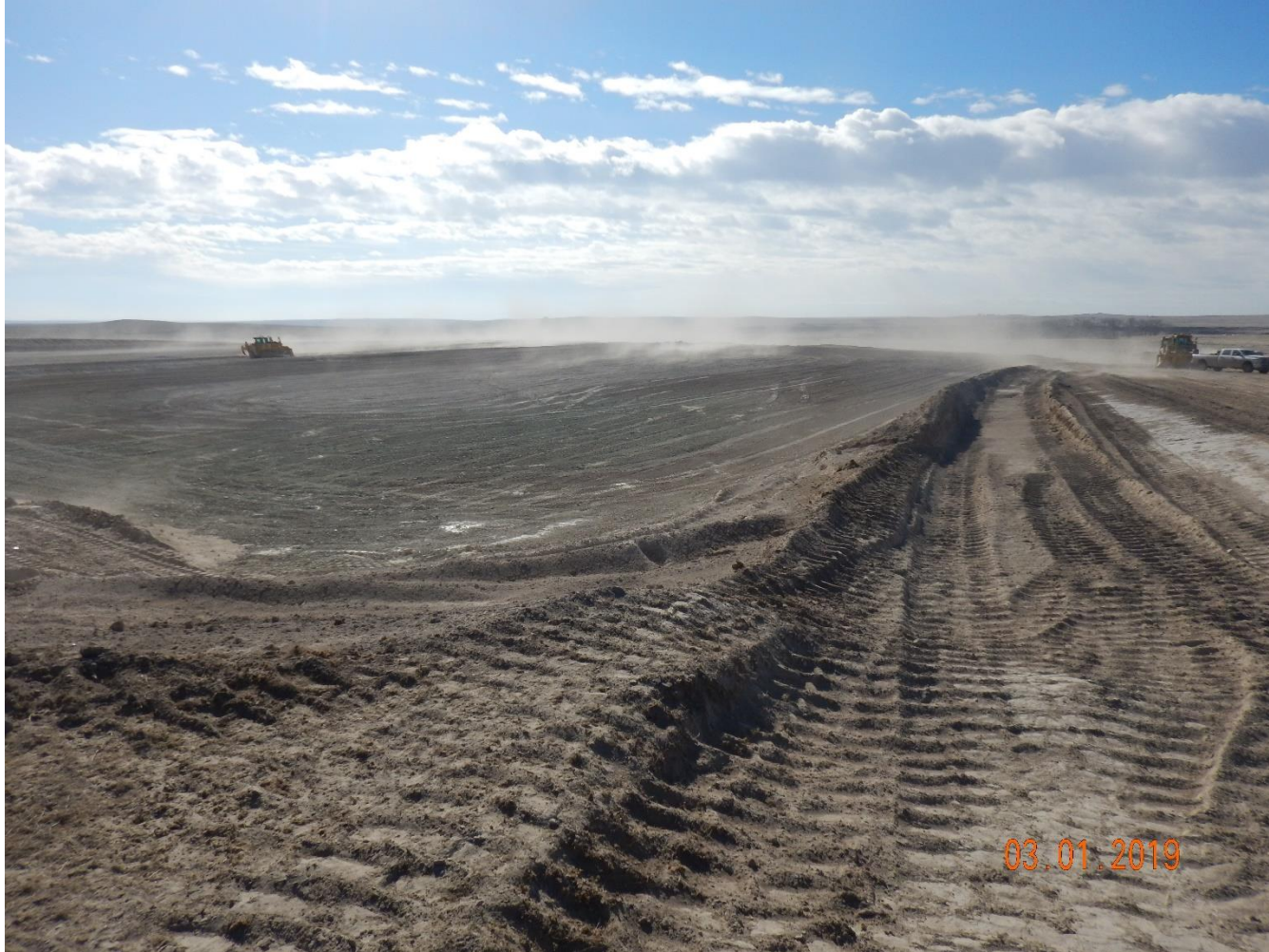
Photo 20: Photo taken from northwest corner of the location, facing southeast. Photo shows ongoing wind erosion degradation transporting sediment off of the location and soil stockpiles.
