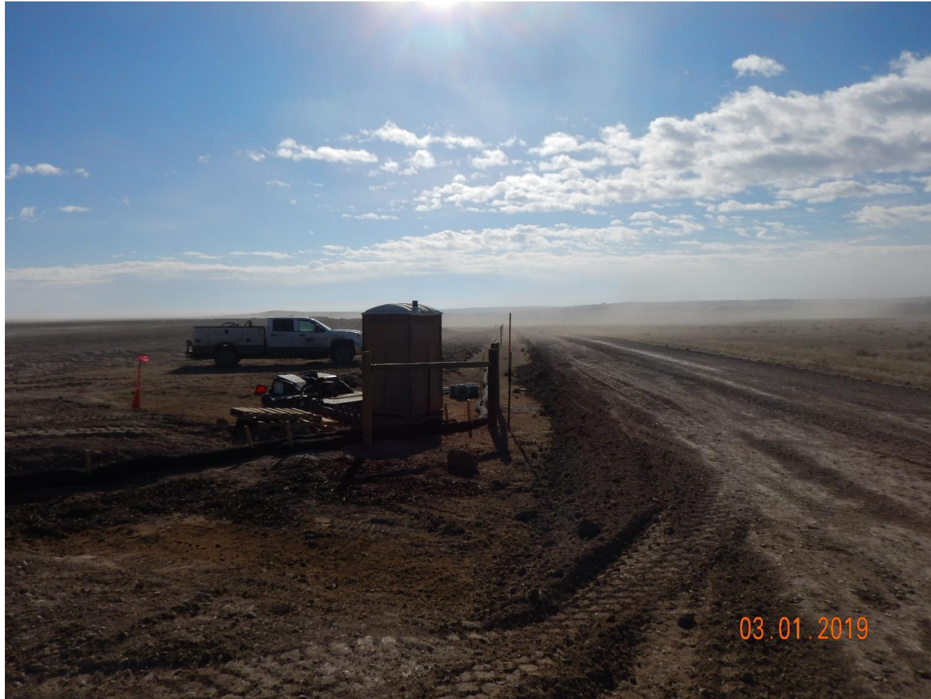
Photo 3: See comment under photo 1. Photo shows ongoing wind erosion degradation transporting sediment off of the location. Operator has failed to implement and maintain sufficient stabilization and erosion control BMPs to mitigate wind erosion and sediment transport on the location in accordance with 1002.f and 1002.e
