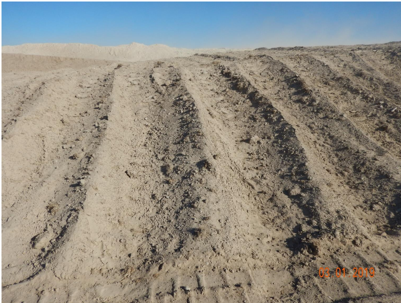
Photo 6: Photo taken from the soil stockpile on the south end of the location. Previous inspection required operator to install BMPs to stabilize the soil stockpiles on location in accordance with 1002.f and 1002.c. Photo shows soil stockpile remains insufficiently stabilized with loose material. Active wind erosion degradation and sediment transport off location occurring on location and soil stockpiles.
