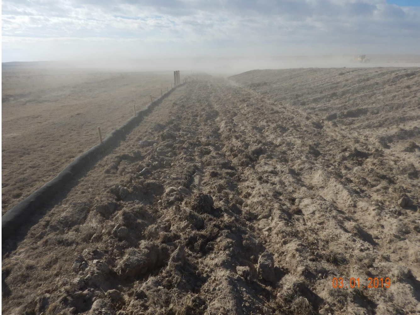
Photo 12: Photo taken from the east end of the location. Photo shows operator appears to have conducted maintenance on the surface roughening BMP per corrective actions. Photo also shows ongoing wind erosion degradation transporting sediment off of the location and soil stockpiles.
