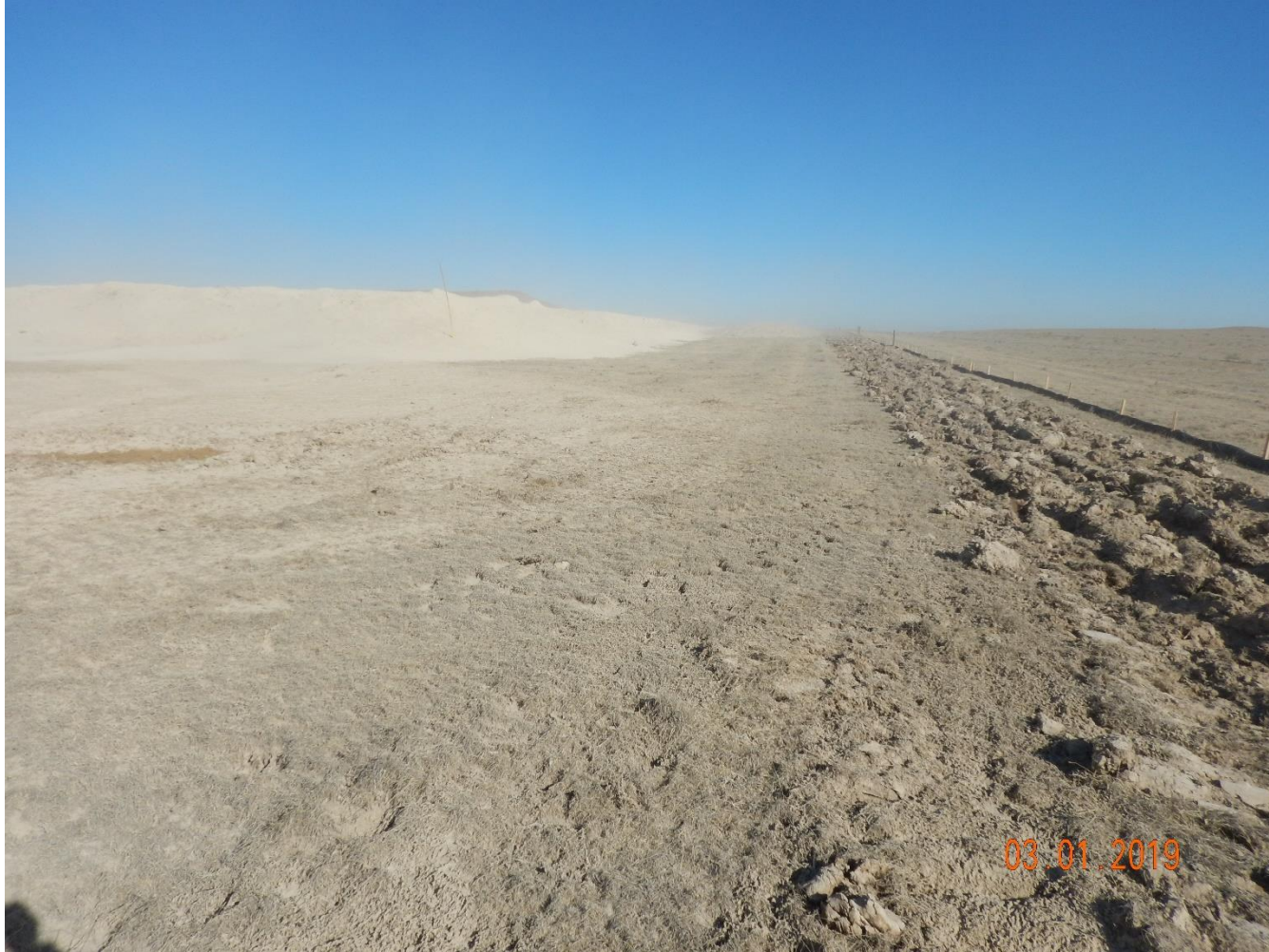
Photo 7: Photo taken from the southeast end of the location, facing north. Photo shows ongoing wind erosion degradation transporting sediment off of the location and soil stockpiles.
