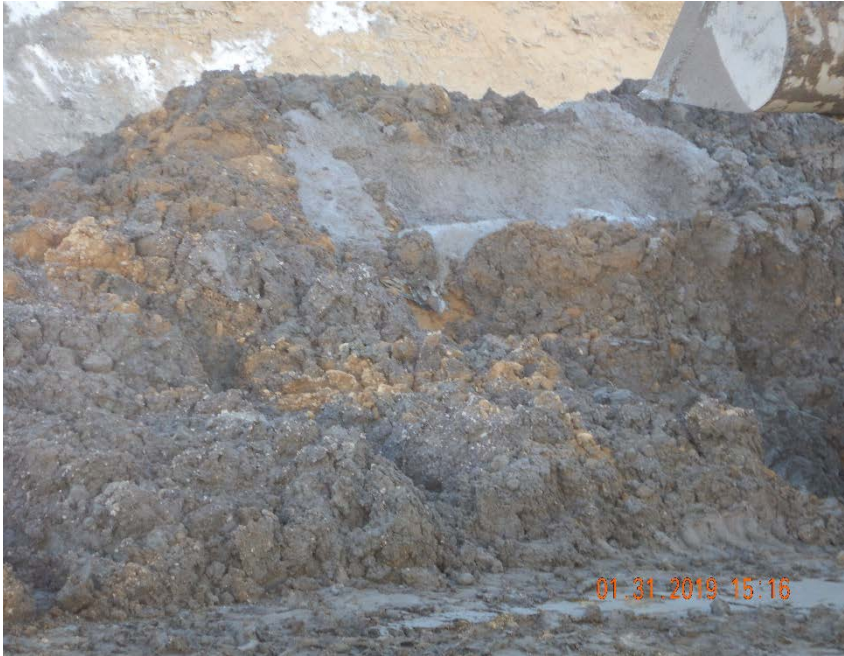
Photo #9 – Fluid accumulations inside of cuttings area. Operator was contacted via phone 1/31/2019 and instructed to comply with cuttings management COAs.
