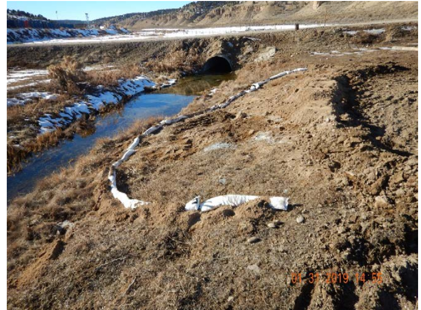
Photo #6 – View of earthen berm and absorbent booms installed at terminus of spill path, looking west. Note proximity to Black Sulphur Creek.
