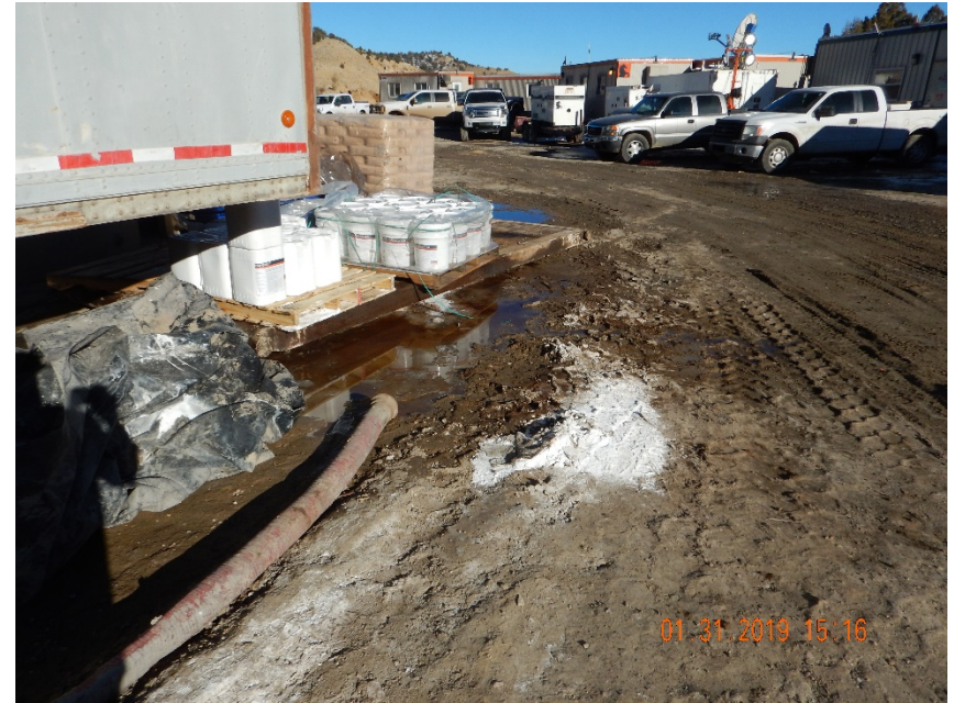
Photo #8 - View of inadequate chemical storage on pad. Operator was contacted via phone on 1/31/2019 and instructed to address spill within 24 hours.
