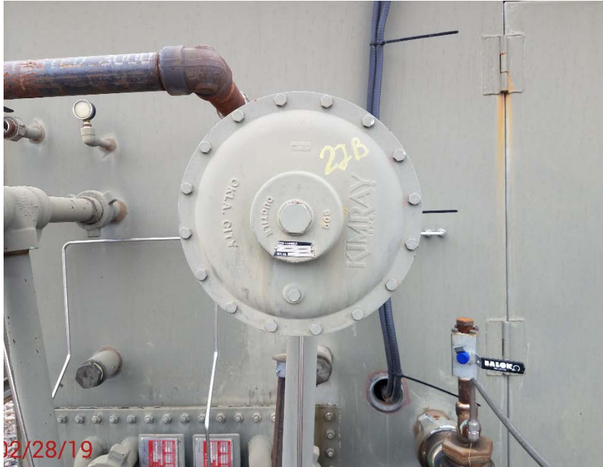
Location Photo #8, Leaking fitting on unit 22B.
