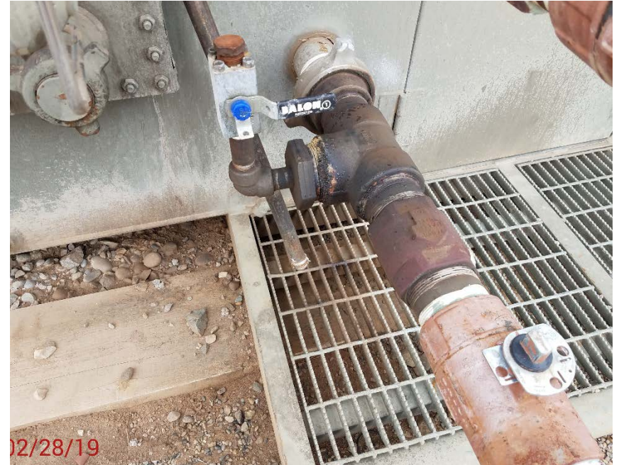
Location Photo #7, Leaking fitting on unit 21B.
