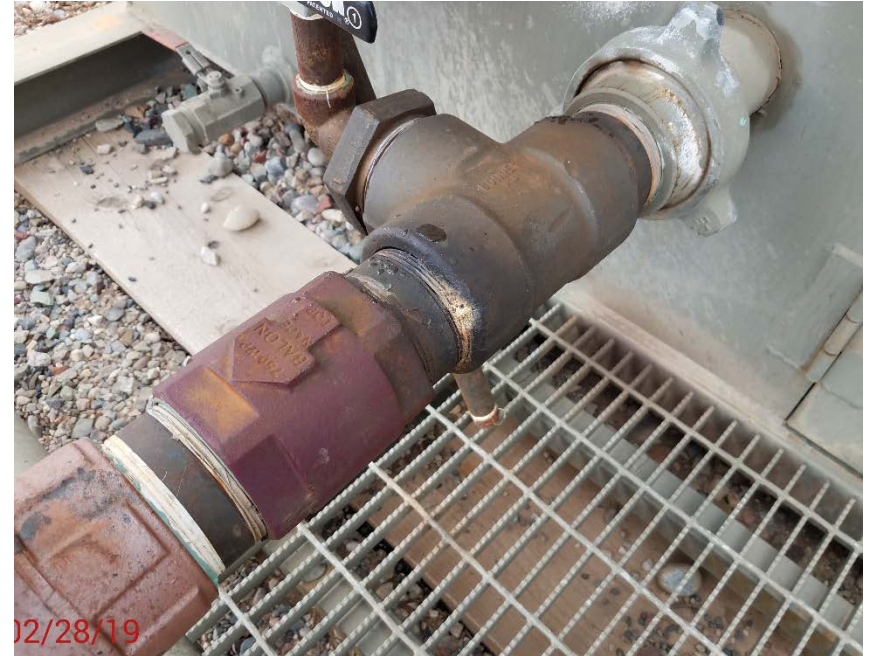
Location Photo #11, Leaking fitting on unit 31C.
