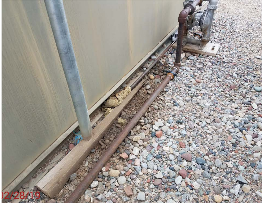
Location Photo #4, stained ground at vent pipe for circulation pump.
