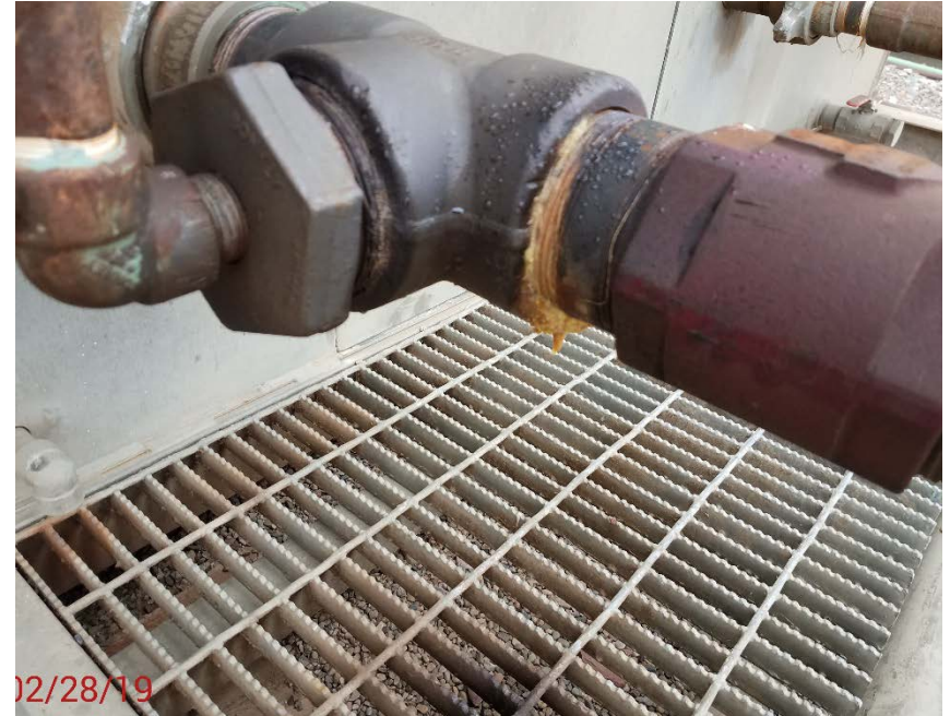
Location Photo #9, Leaking fitting on unit 22B.
