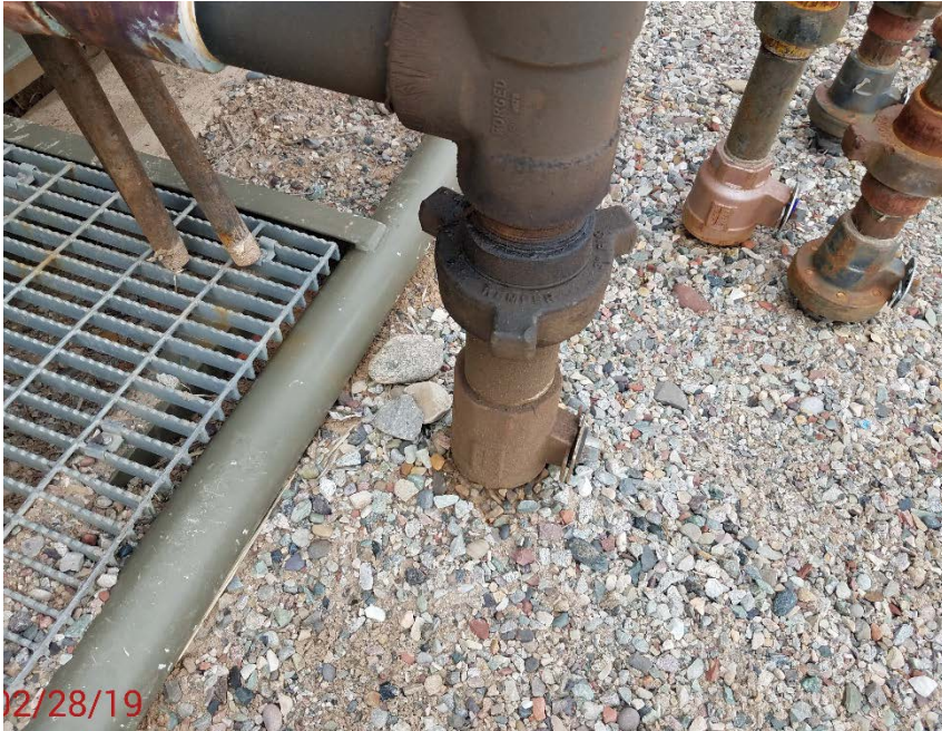
Location Photo #11, 2 of 2 Leaking fitting on unit 23A.
