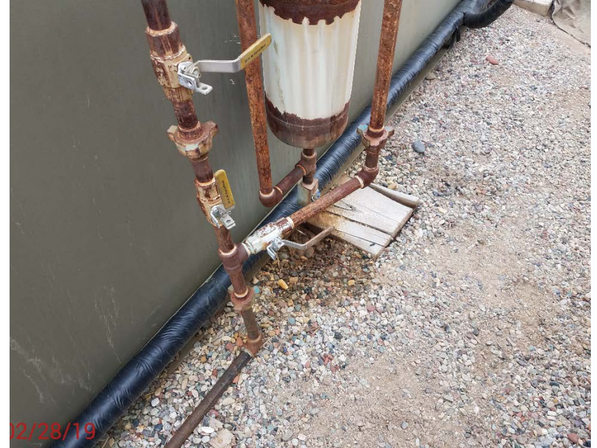
Location Photo #6, Stained ground underneath scrubber pot.
