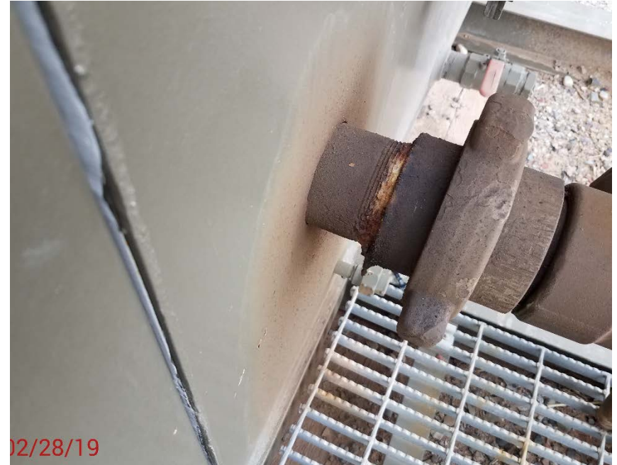
Location Photo #10, 1 of 2 Leaking fitting on unit 23A.
