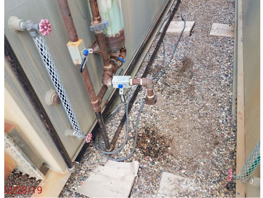
Location Photo #8, Stained ground underneath scrubber pot.
