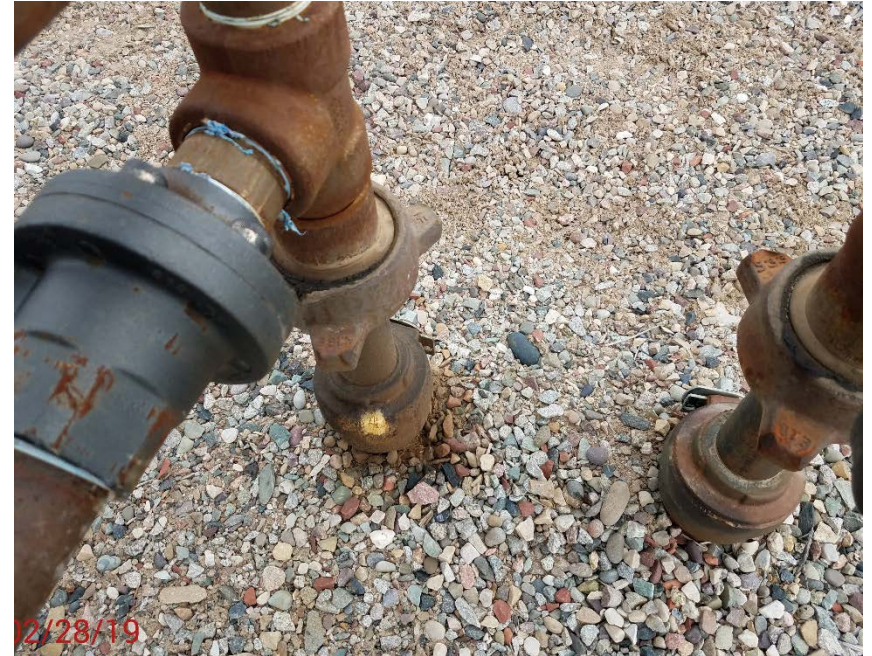
Location Photo #13, leaking fitting on 24D.
