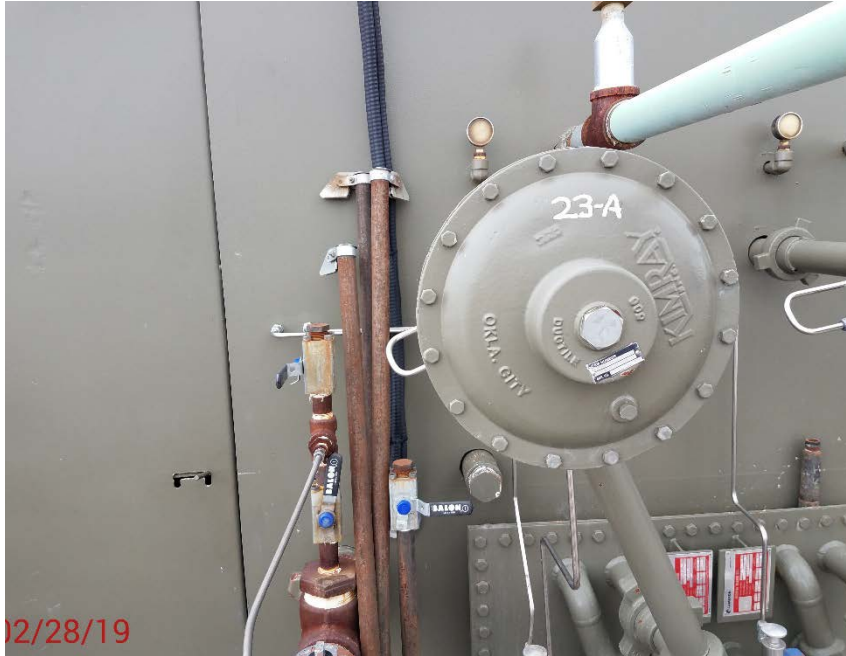
Location Photo #9, 2 Leaking fittings on unit 23A.
