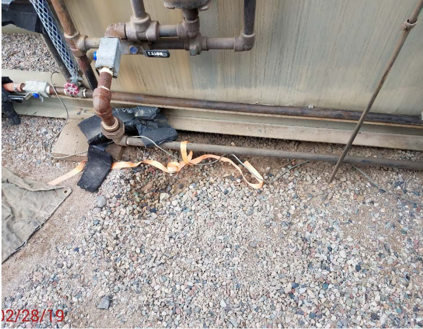
Location Photo #7, Stained ground underneath scrubber pot.
