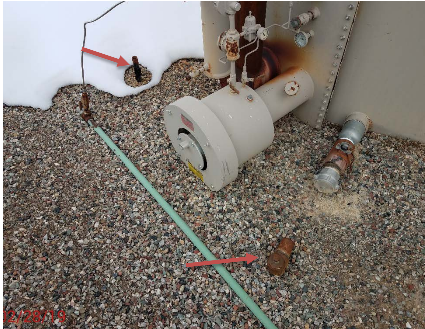
Location Photo #3, 2 unmarked/unused flowline risers in tank battery.
