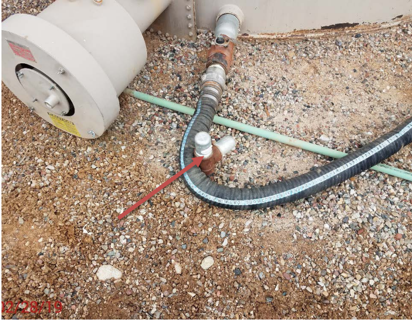
Location Photo #5, 1 unmarked/unused flowline risers in tank battery.
