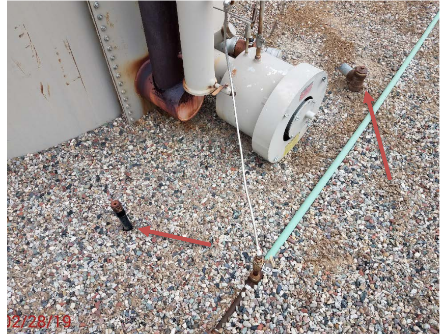
Location Photo #4, 2 unmarked/unused flowline risers in tank battery.
