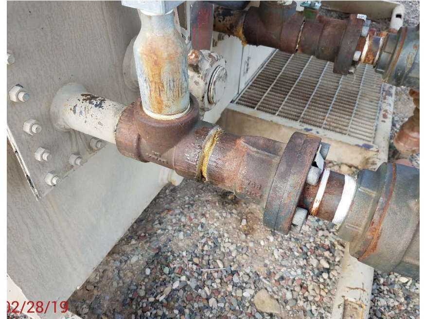
Location Photo #6, leaking fitting on inlet flow line.
