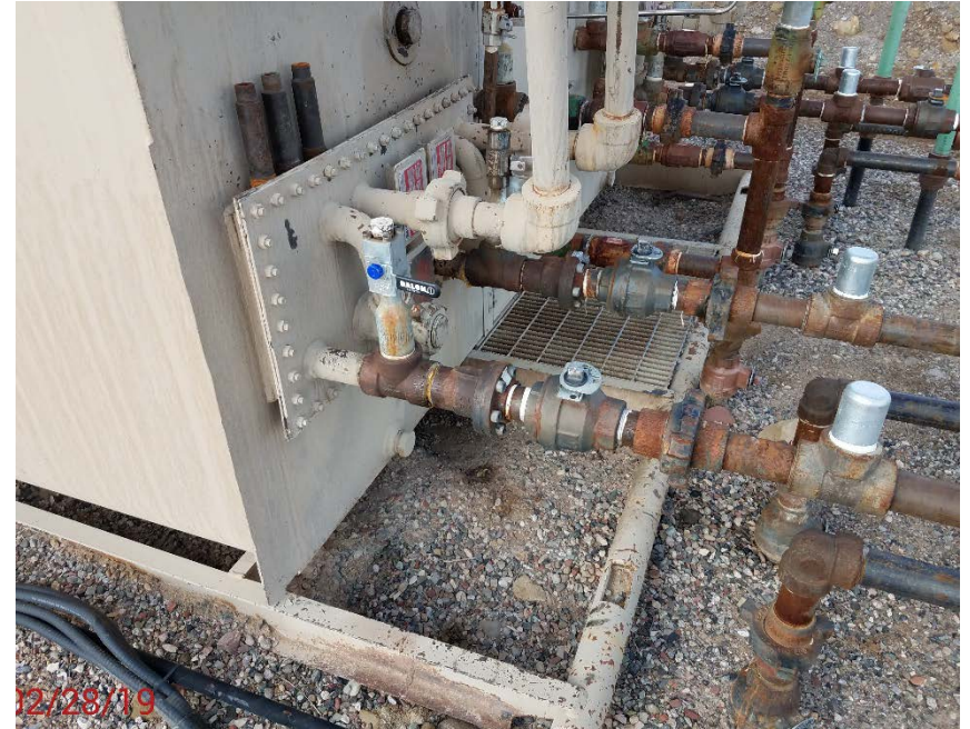
Location Photo #4, 2 leaking fittings on inlets to separator.
