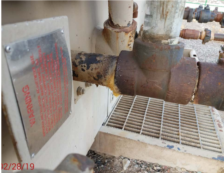
Location Photo #5, leaking fitting on inlet flow line.
