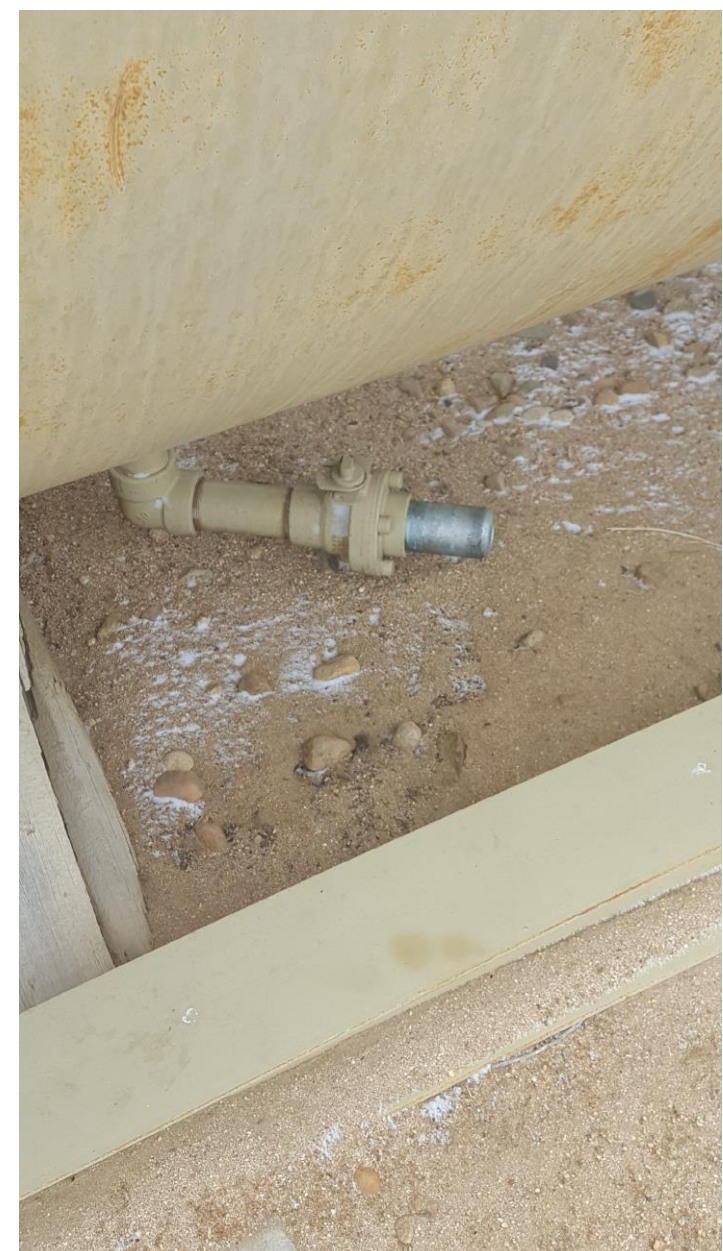
Figure #1 Bull plugs have been installed.
