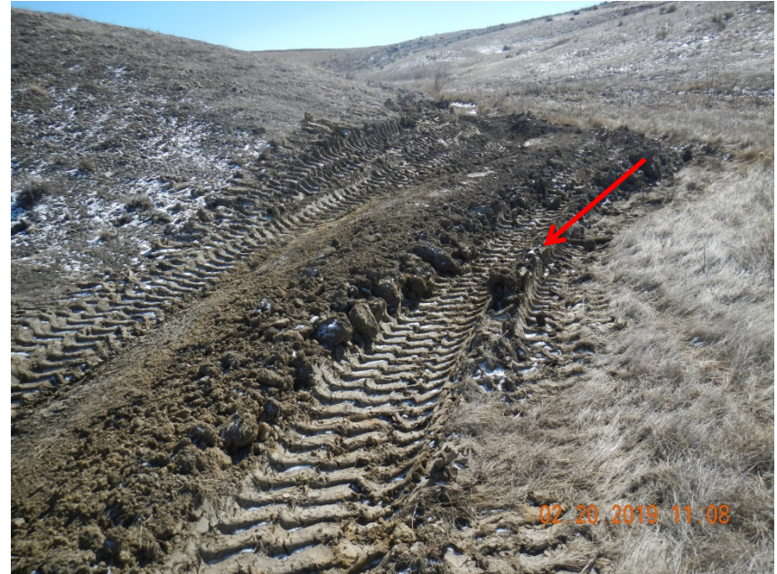
Photo 12. Photo taken from the southwestern perimeter of the location, facing East. Photo illustrates the ditch and berm BMP that has been improperly installed, not compacted and has been disturbed due to equipment.
