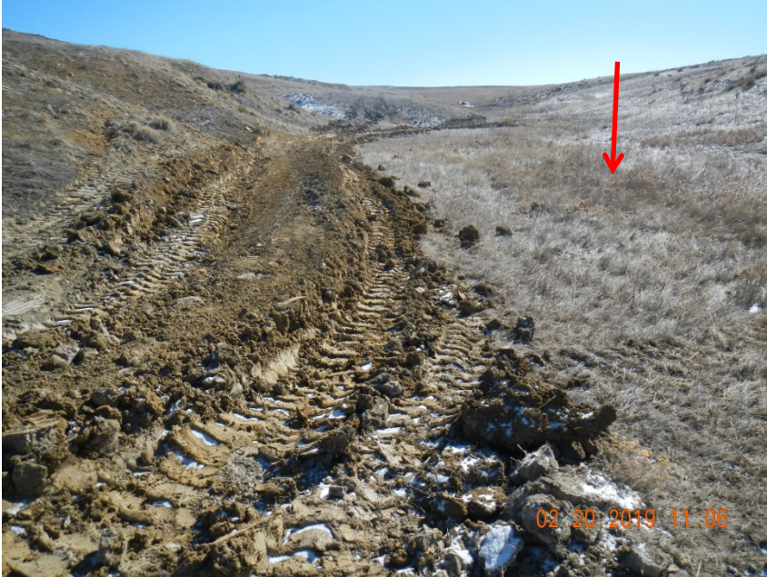
Photo 13. Photo taken from the southern perimeter of the location, facing East. This entire southern perimeter is a USFWS National Wetlands Inventory mapped Riverine System (R4SBC) wetland and has been disturbed due to the construction.
