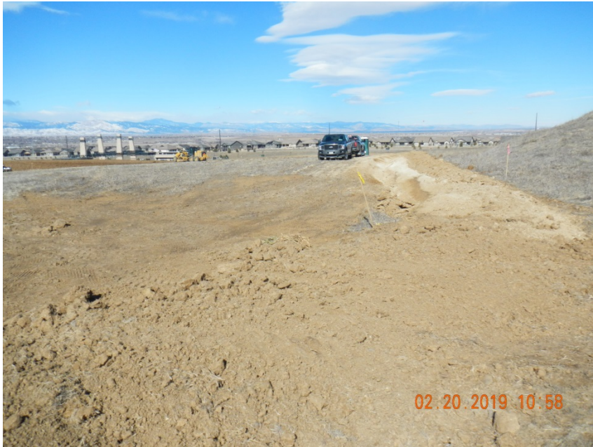
Photo 1. Photo taken from the eastern perimeter of the location, facing North. Photo illustrates a ditch and berm BMP that is being installed around the perimeter of the location. However this should have been complete at the time of inspection because major dirt work activities were occurring at the center of the location.
