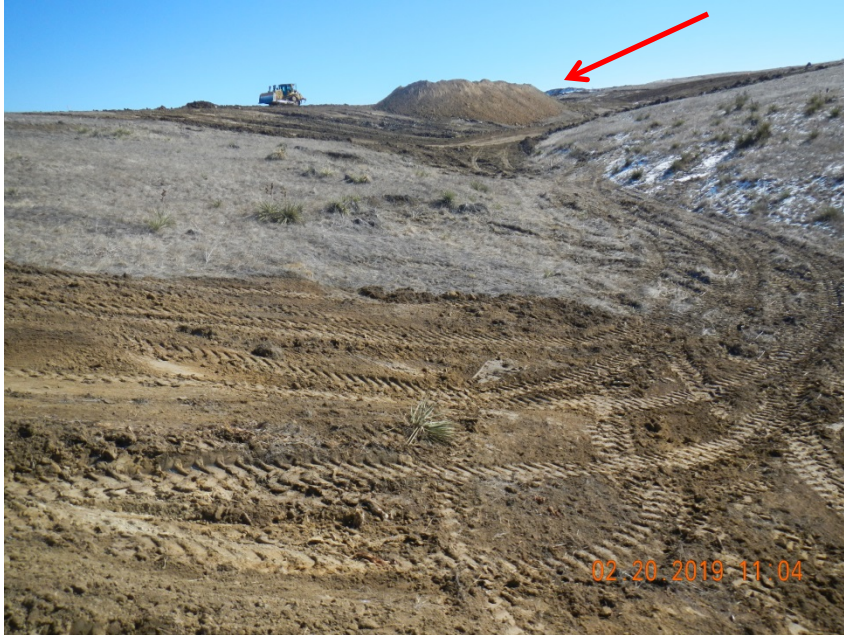
Photo 9. Photo taken from the western perimeter of the location from where the break in the ditch and berm BMP is located, facing East. Note the upslope work being conducted at the time of the inspection there were no BMPs downslope of the construction.
