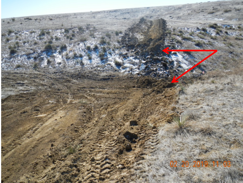
Photo 7. Photo taken from the western perimeter of the location, facing South. Photo illustrates the ditch and berm BMP was not completed at the time of inspection. Note there is a potential wetland downslope within the drainage where the break in the ditch and berm BMP is located.
