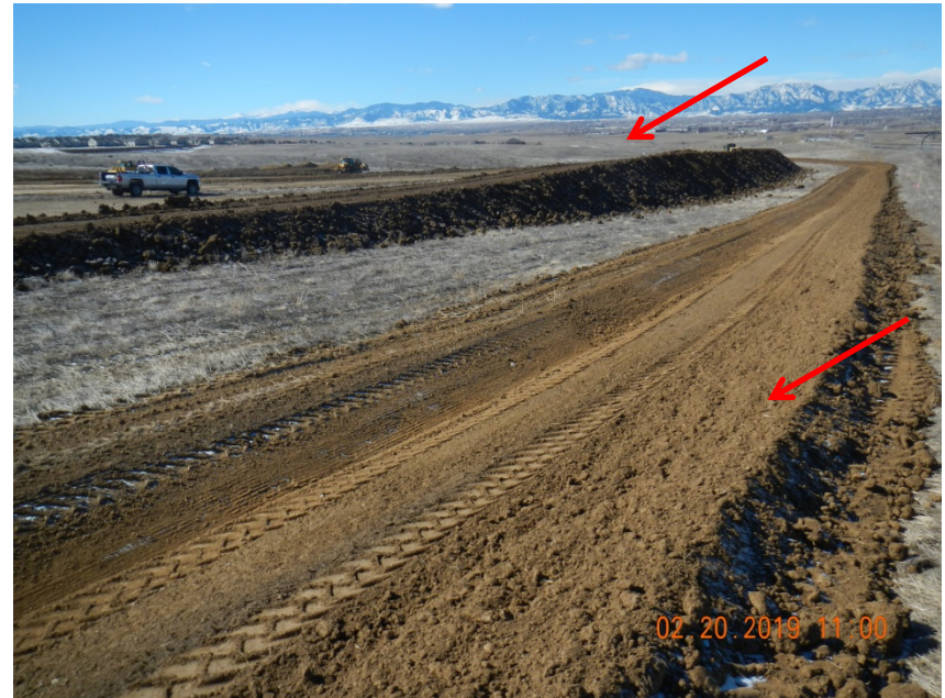
Photo 4. Photo taken from the northeastern perimeter of the location, facing West. The topsoil stockpile being stored along the northern area in the background of the Photo. The perimeter BMPs in the foreground of the Photo have not been completed due to lack of compaction and has not been installed with best engineering practices. However this should have been complete at the time of inspection because major dirt work activities were occurring at the center of the location.
