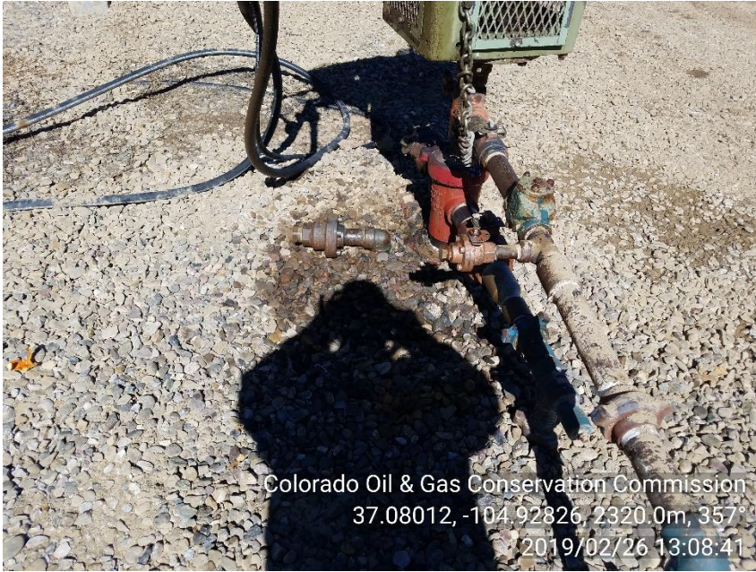
PHOTO 3: STAINED SOIL UNDER DRIVE HEAD MOTOR
