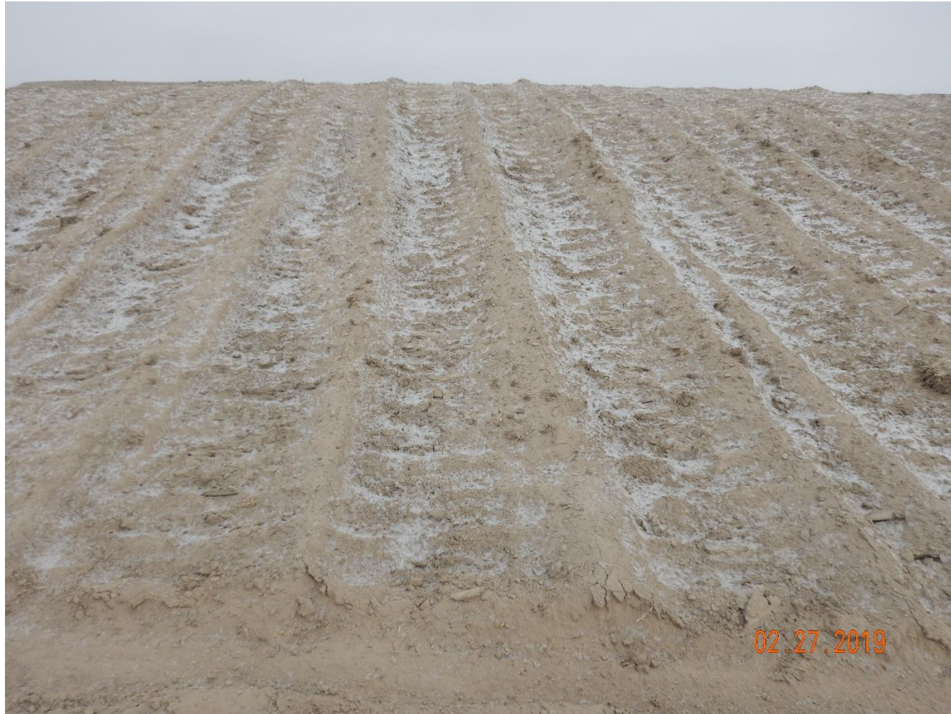
Photo 10: Continued from photo 9. Photo shows operator appears to have attempted to track the soil stockpile. Photo shows tracking does not appear to have been adequate as soils have not been sufficiently stabilized and remain loose material at risk to erosion degradation.
