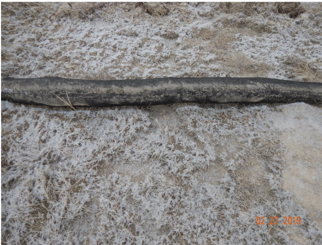
Photo 18: Photo shows Operator has installed an 8 inch diam. "Filtrexx SiltSoxx" wattle as a perimeter control. Operator has installed BMP by placing wattle upon the surface of the soil and staking in place. The following photos are examples that show that due to site conditions found commonly within rangeland (bumpy, rocky, changes in elevation affecting ground surface contact), this "lay on surface" installation practice is not appropriate or sufficient to allow this perimeter control to mitigate stormwater runoff on rangeland; BMP does not achieve a 100% ground surface contact to interrupt and mitigate stormwater runoff.
