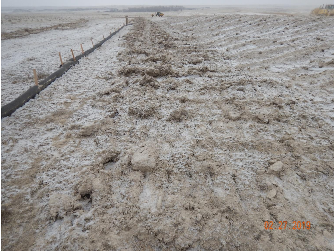
Photo 16: Photo taken from the east end of the location. Photo shows operator appears to have driven over the surface roughening BMP along the perimeter of the location. BMP is no longer in proper functioning condition and requires maintenance.
