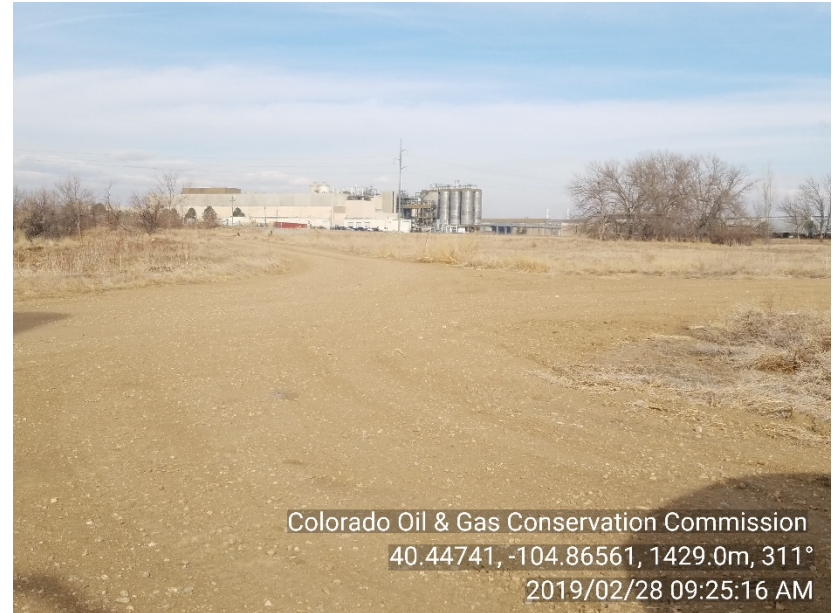
Photo #16 Great Western 35-52 Access Road Ruts Appears mitigated
