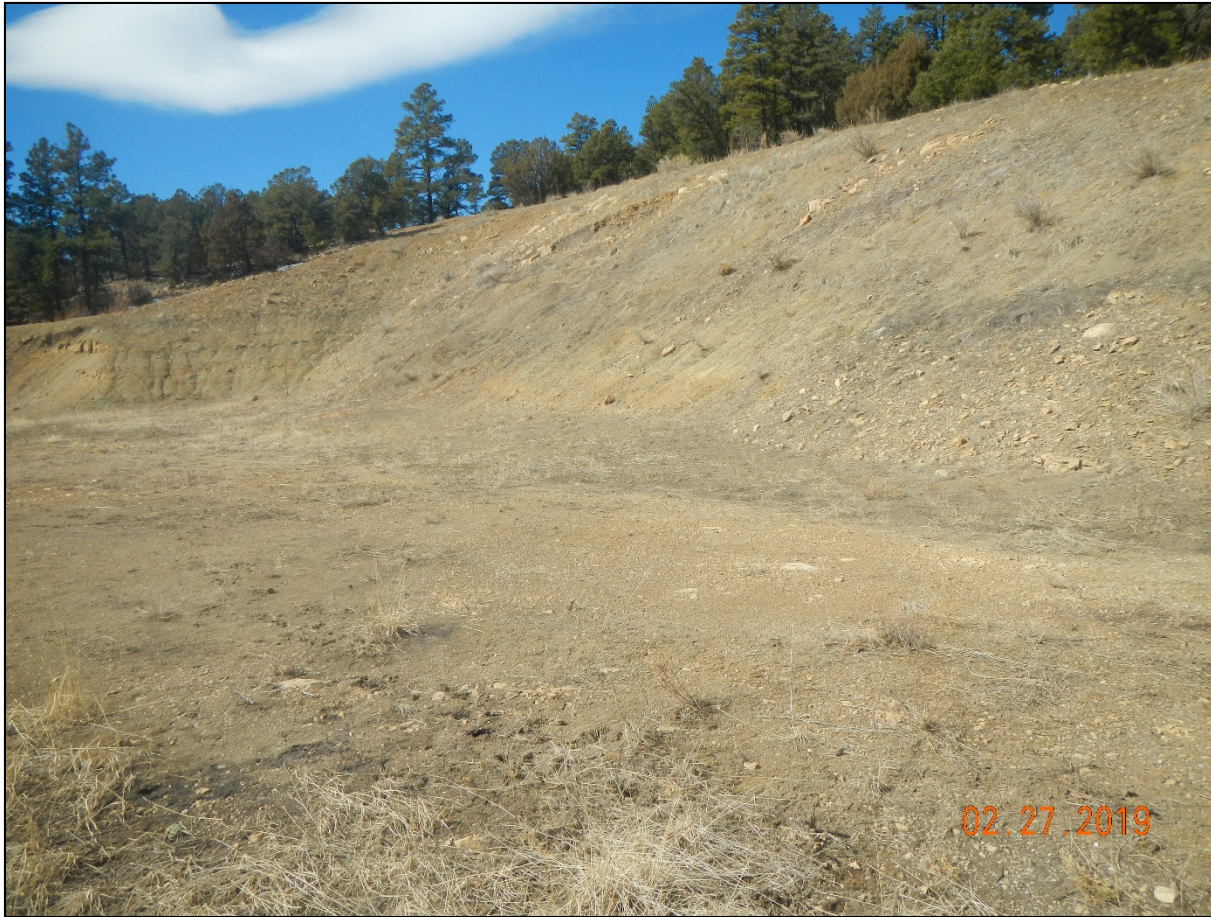
Photo 9. East side of the location facing toward the cut slope. The cut slope is not stabilized with vegetation. There are signs of soil sloughing and erosion.
