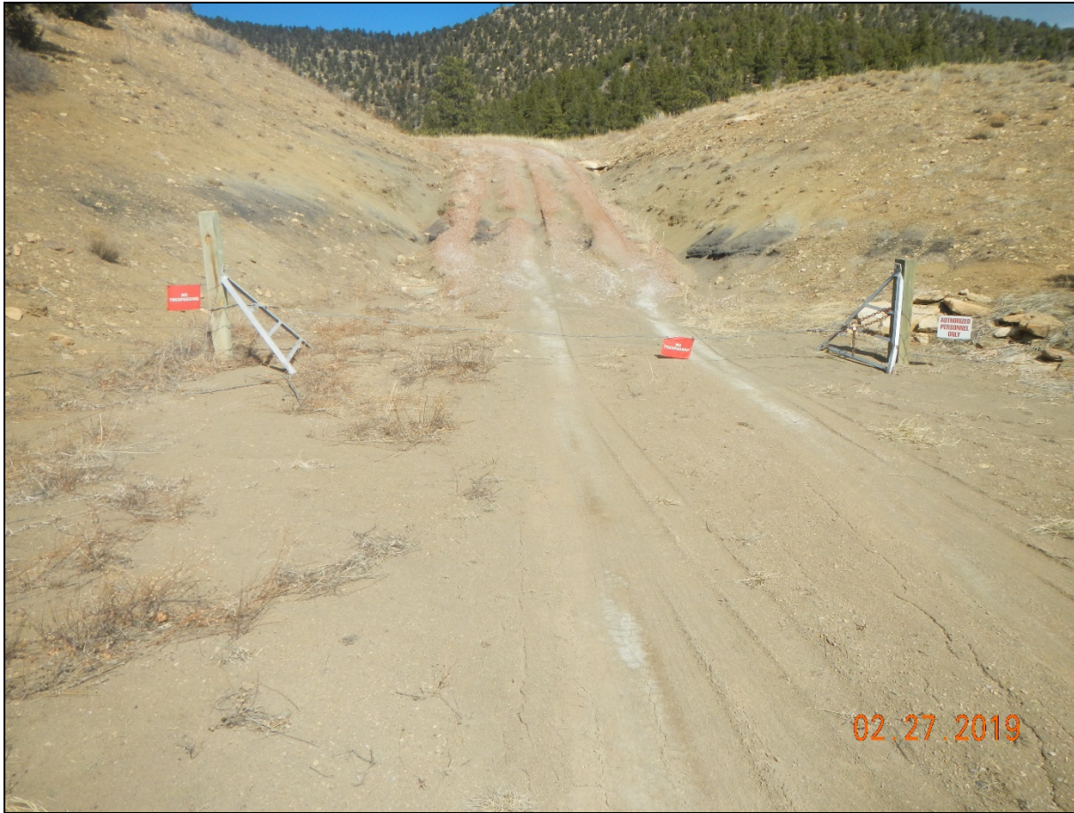
Photo 1. Facing north at the beginning of the access road. Sediment has filled in the cattle guard and is being deposited in the roadway.
