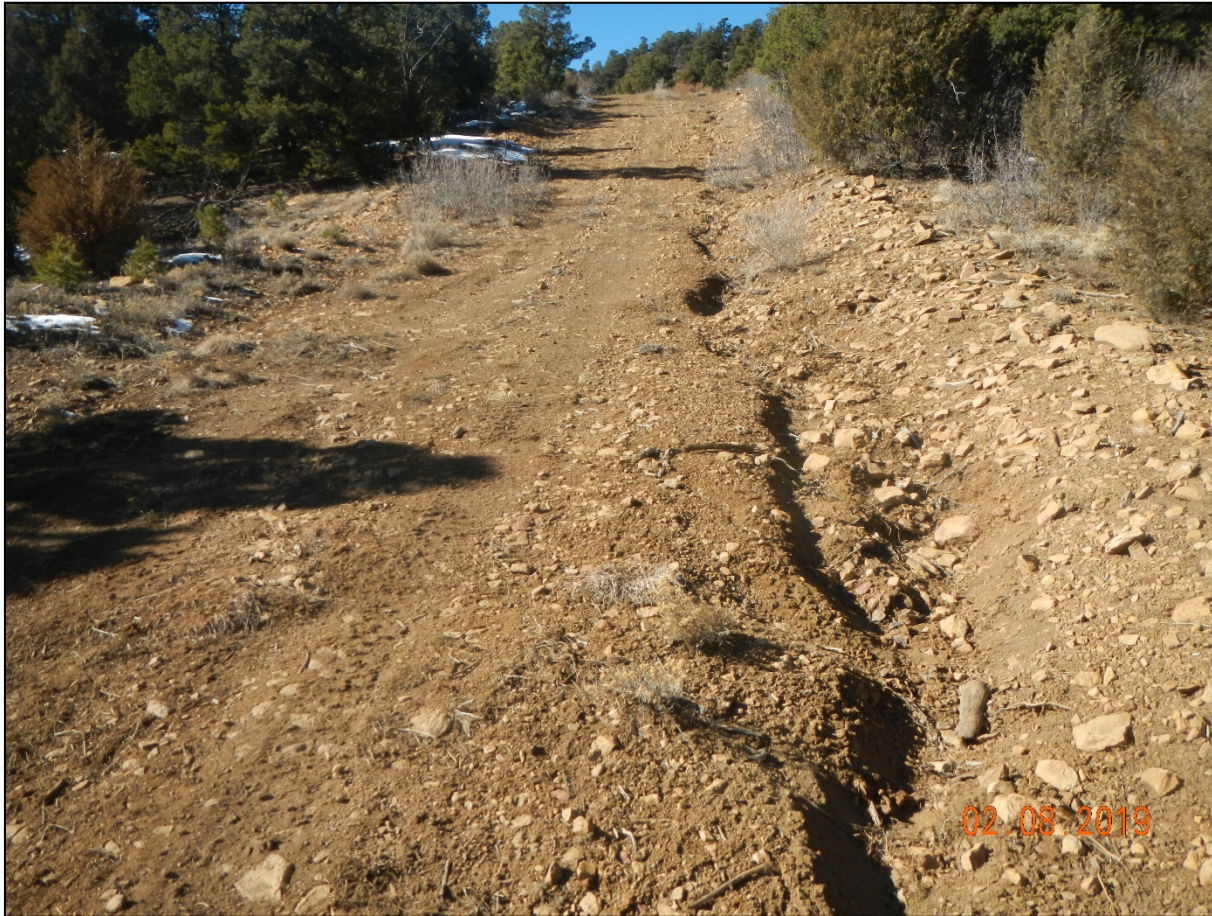
Photo 4. Erosion is occurring on the side of the road and there are no BMP's.
