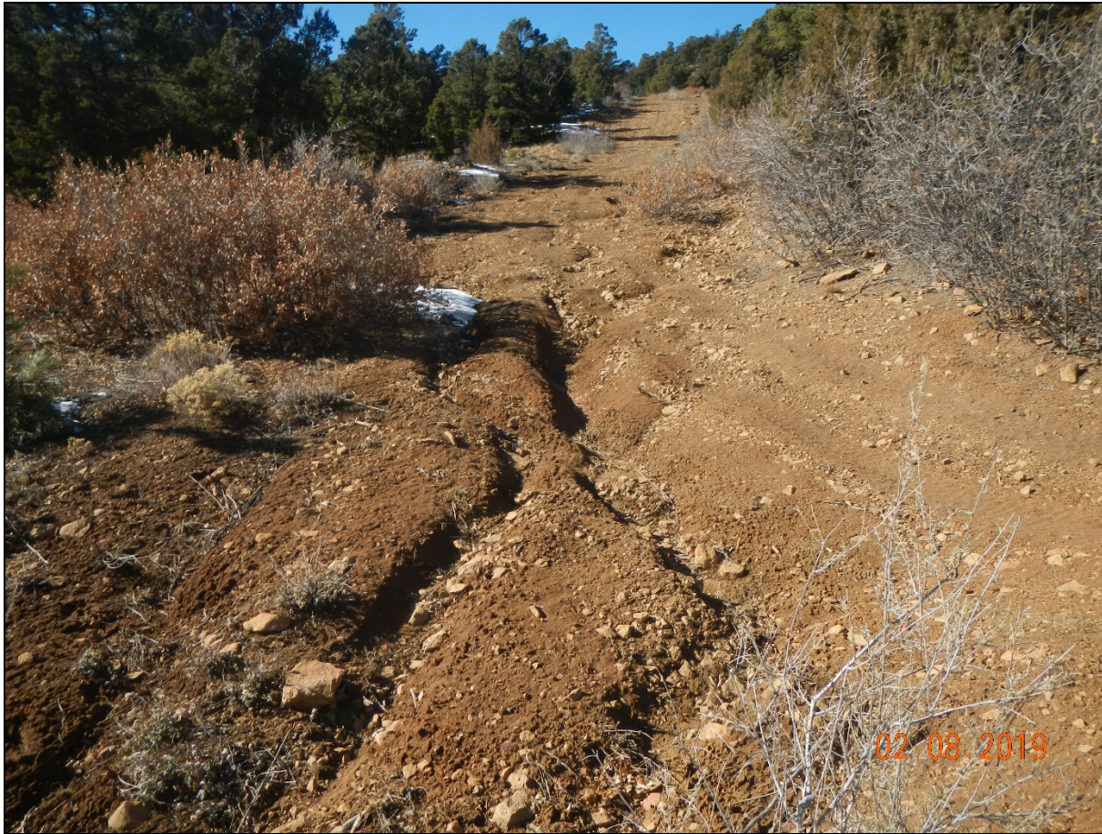
Photo 3. There are signs of erosion occurring along areas of the access road.
