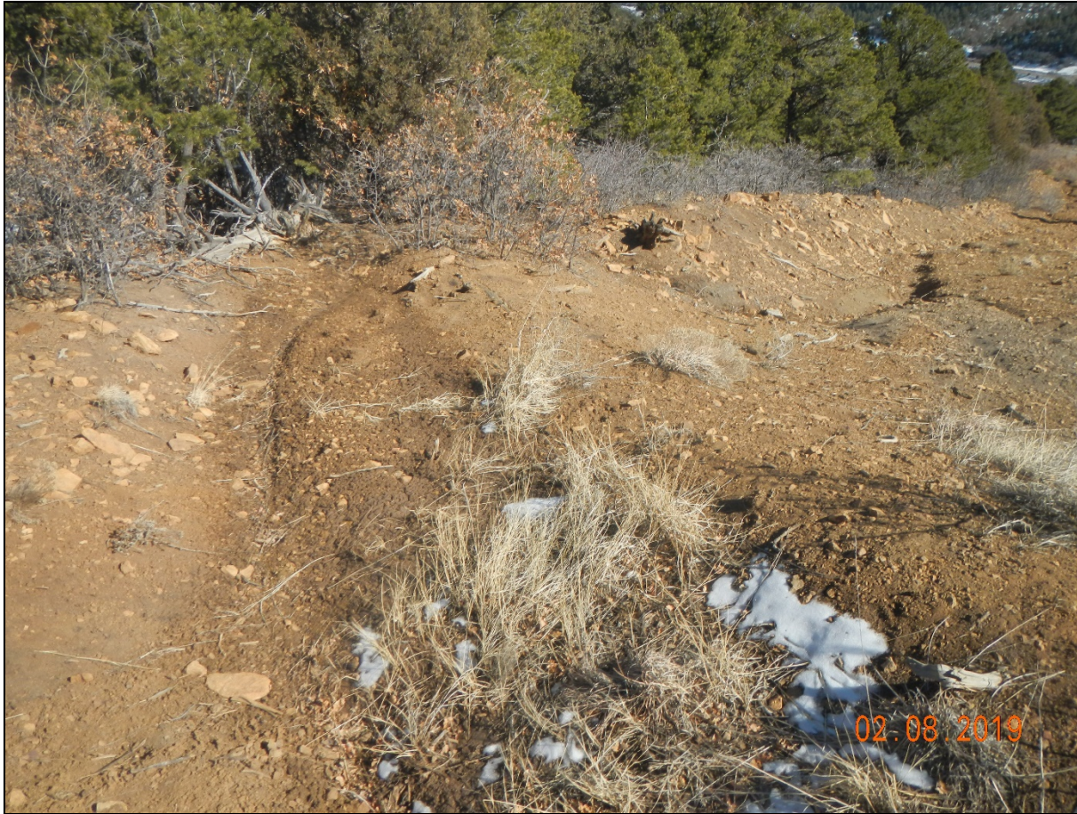
Photo 5. This water bar is filled in with sediment and stormwater is directed back toward the road.
