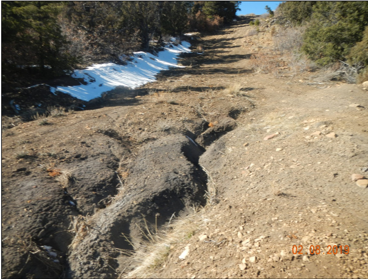
Photo 6. Further along the road near the location. There is erosion rills developed along the road.
