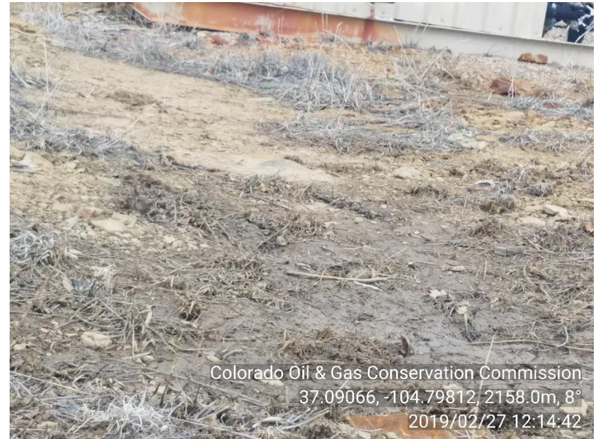
PHOTO 6: MORE WET SOIL OUTSIDE METER HOUSE. IT APPEARS THAT FLUID FROM SEPARATOR IS BEING DRAINED ON THE GROUND.
