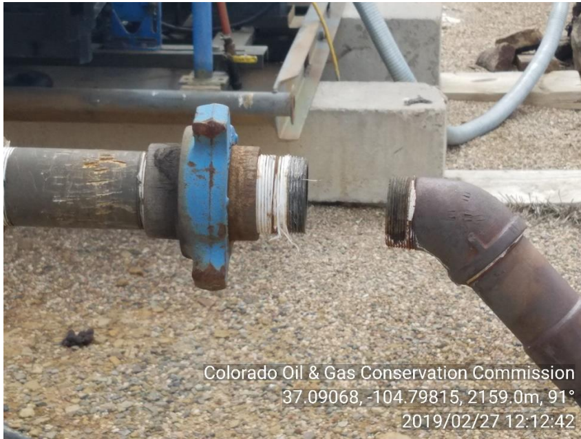
PHOTO 3: VALVE MISSING.
