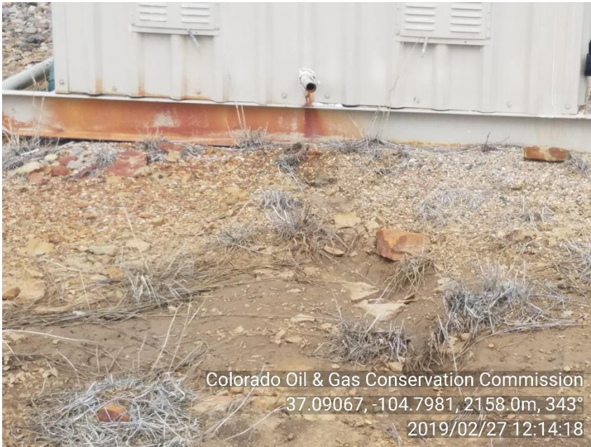
PHOTO 5: WET SOIL OUTSIDE METER HOUSE. IT APPEARS THAT FLUID FROM SEPARATOR IS BEING DRAINED ON THE GROUND.
