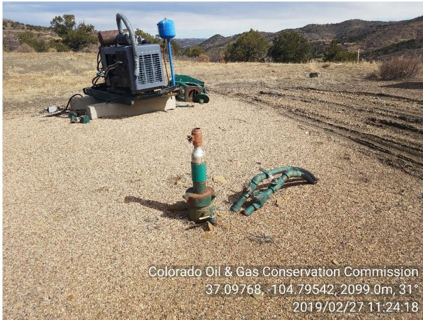
PHOTO 3: TWO UNMARKED UNUSED RISERS NO LOTO/CASING NOT LO/TO.
