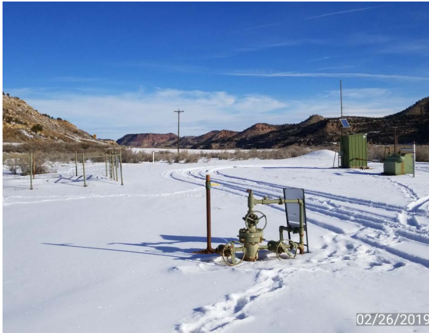
Photo 1. Location looking north.
