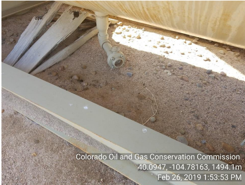
Photo 13 no bull plug on drain line of separator
