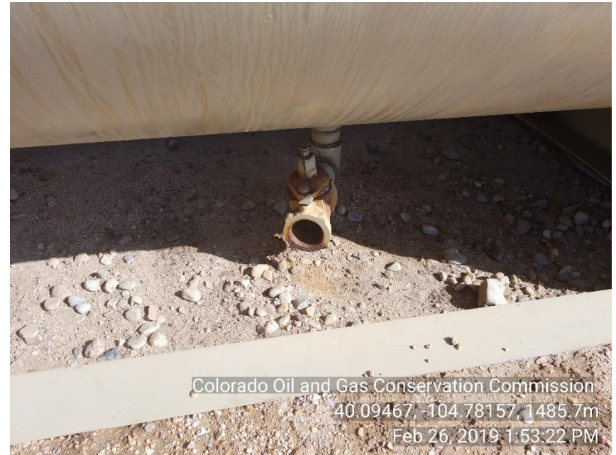
Photo 12 no bull plug on drain line of separator
