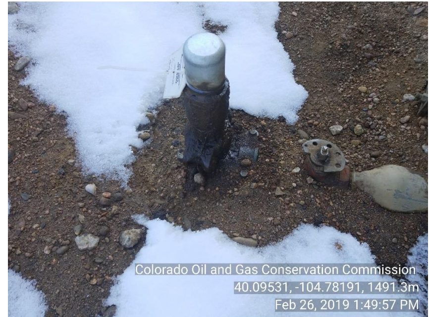
Photo 8 stained soil 2" bull plug on crude oil load line to tank
