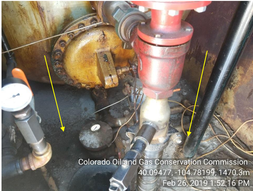
Photo 11 Stained soil inside separator house
