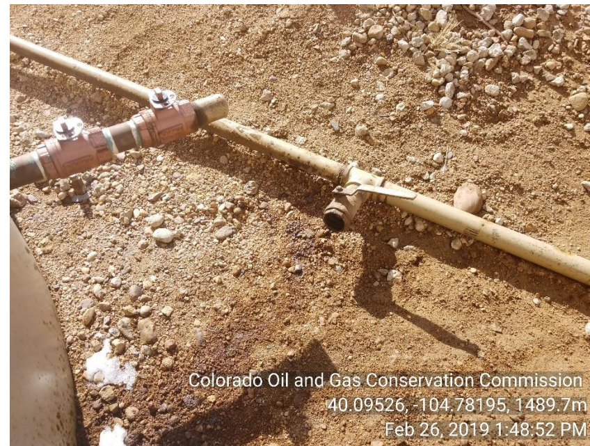
Photo 6 Stained soil under disconnected crude oil load line and no bull plug on 2" VLV
